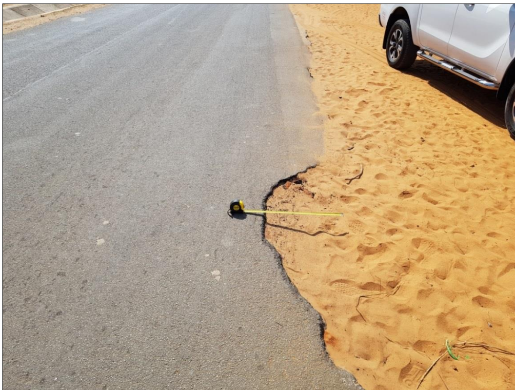
Figure 29: R241 – Edge cracking and erosion
