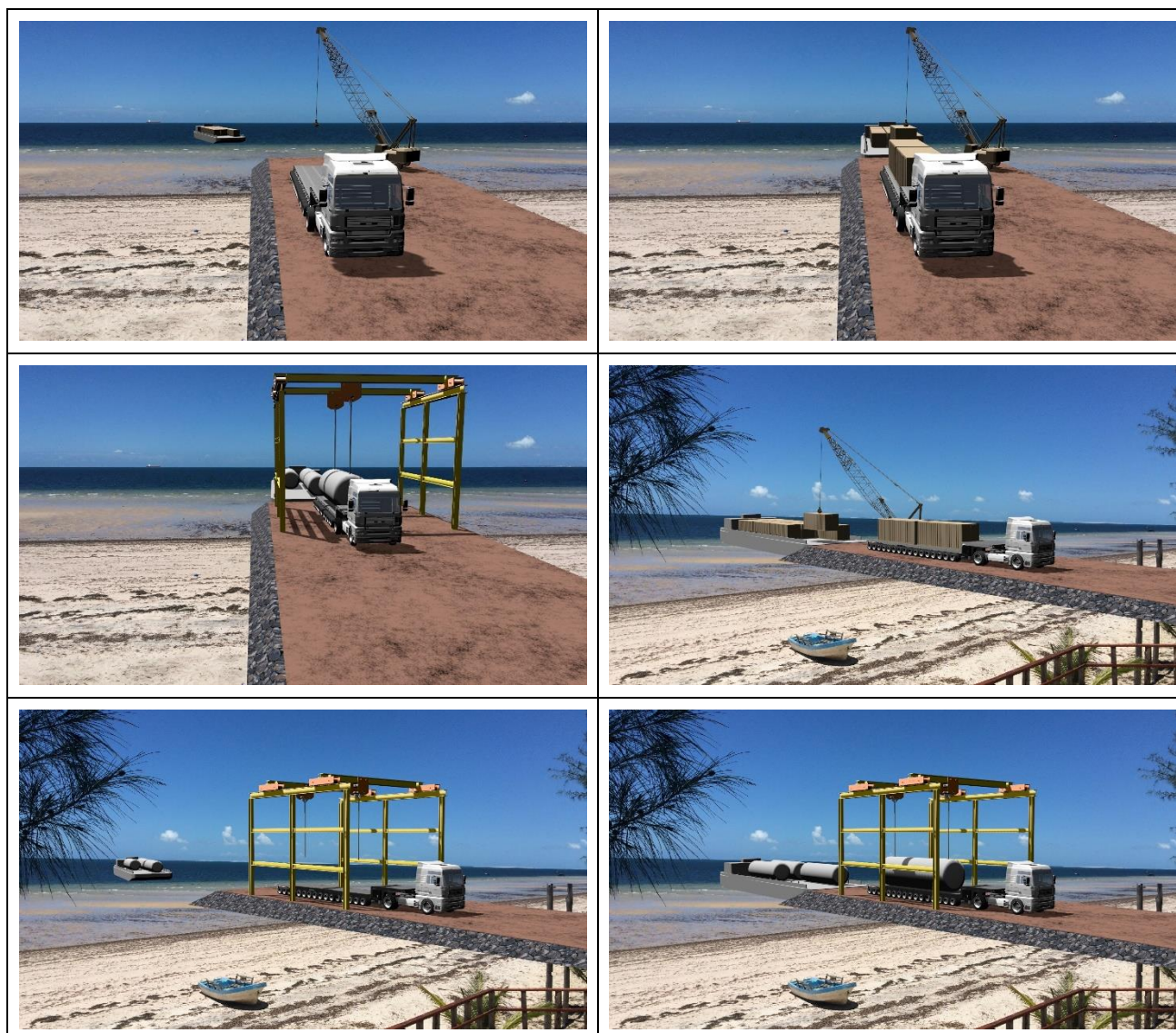
Figure 23: SETA beach landing site during various phases of equipment and material offloading
