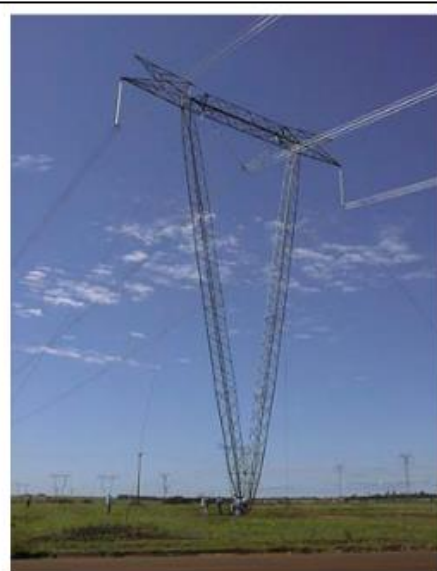
SUSPENSION TOWER - GUYED V TOWER
