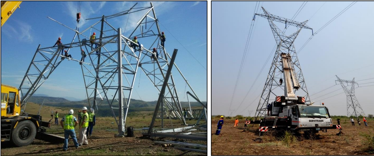
Figure 12: Examples of Pylon construction (source: http://csccon.co.za/ and EDM)
