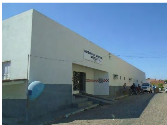
Photo 5.3-11 – Municipal maternity hospital in São João do Piauí.
