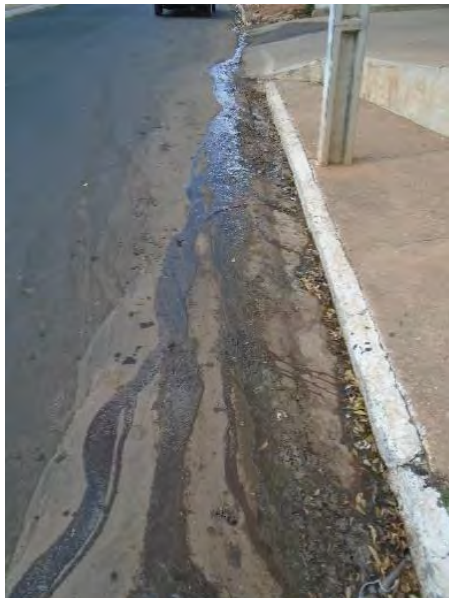
Photo 5.3-13 – open-air sewage discharge at the headquarters of Capitão Gervásio Oliveira (02/11/2016).
