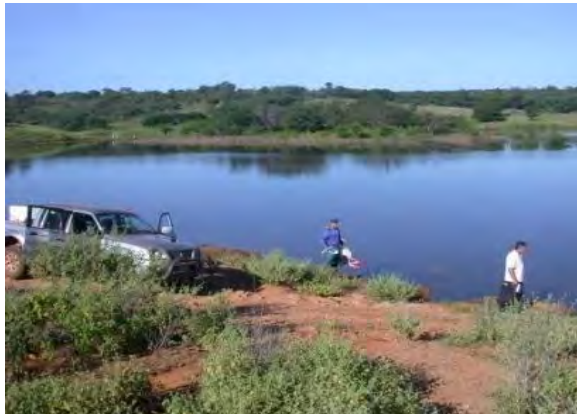
Photo 5.1-57 – View of the Várzea weir (3 rd campaign).
