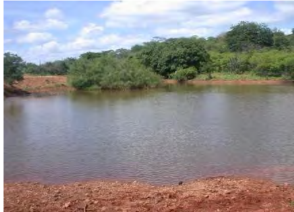
Photo 5.1-60 – View of the weir (3 rd campaign).
