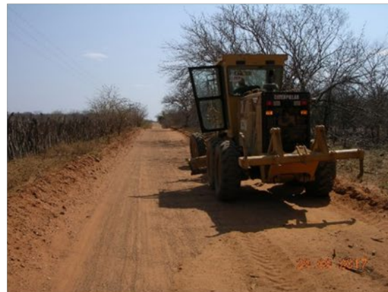
Road that connects the Demo Plant (and PNP1000) to the PI-465 (east), being repaired by municipality.
