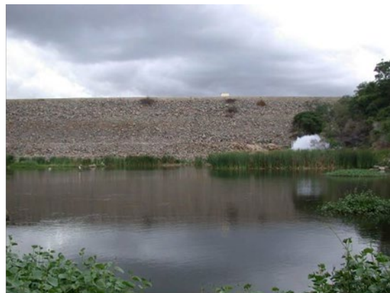
Sampling site 6, view of the spillway of the Jenipapo Dam, Piauí river.
