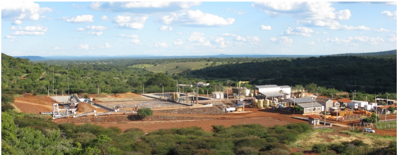
Figure 4-11 BRN’s Piauí Nickel Demonstration plant
