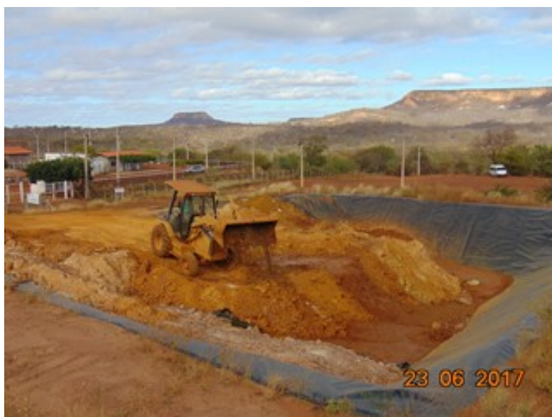
Figure 4-25 Disposal in an Impermeable Residue Storage Area of Solid Demonstration Plant Residues
