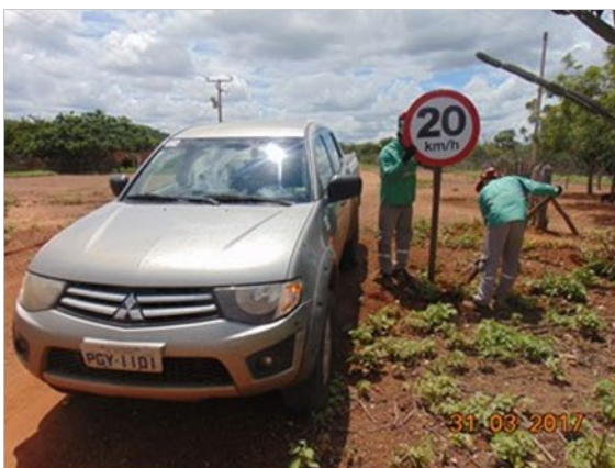
PNM supporting signaling improvements in the ADI's local road.
