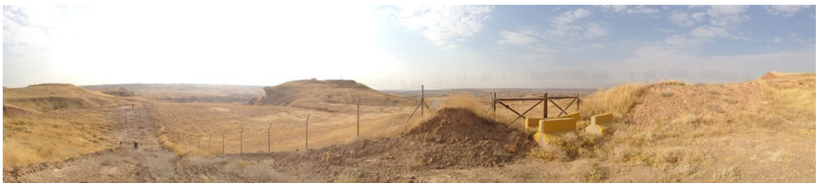
Figure 3-13 Khor Mor perimeter fence at coordinate 35.143803°(N), 44.815793° (E)
