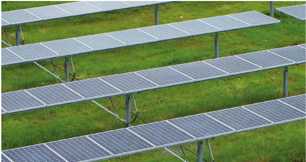
Figure 5 Mounted 1-axis tracker PV (example)
