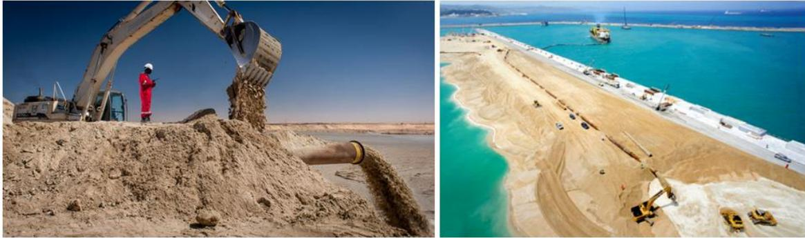
Figure 2-2: Example of bund construction by pumping dredged material from TSHD ashore [B.3]
