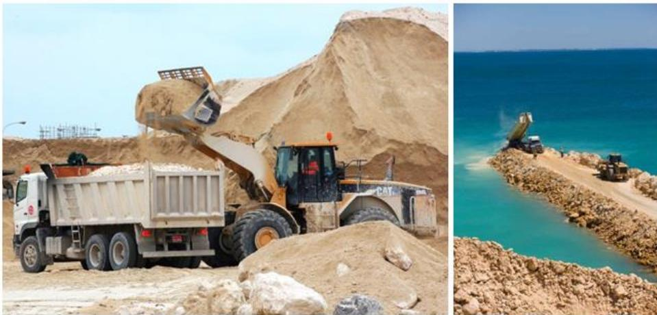
Figure 2-3: Example of bund construction by dump trucks [B.3]
