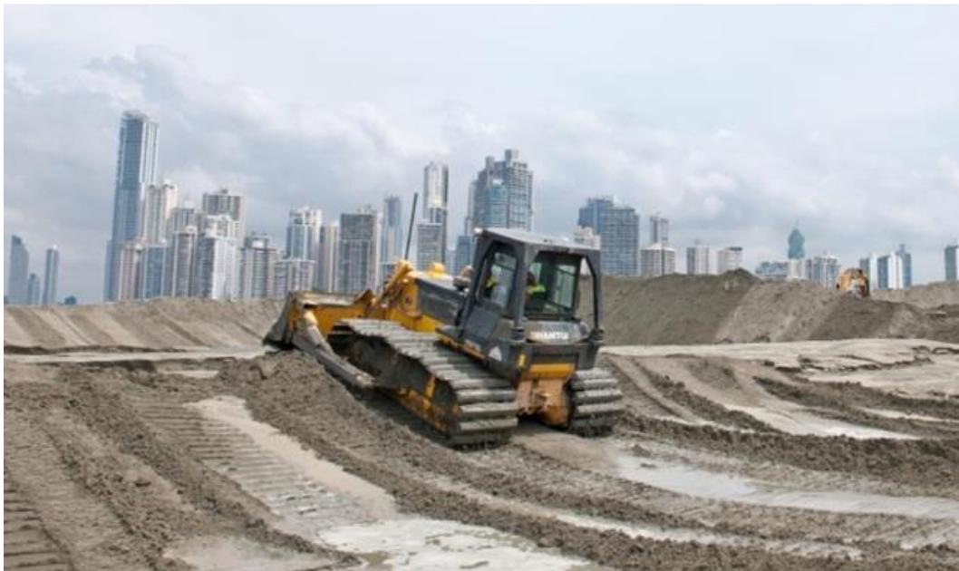
Figure 2-5: Example of a bulldozer leveling a disposal area
