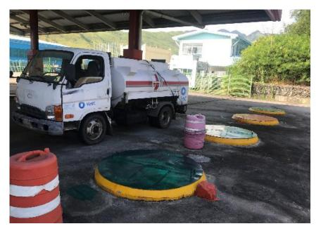
There are reportedly 4 USTs that can be reached via the entry hatches at the gasoline station (right). No spills were detected near the UST. Only calibration records of the tank were received, but no actual maintenance records or a permit for operation. Calibration records of 2009 show that the tank sizes are respectively 16,882, 27,913, 27,768 and 28,042 liters.
