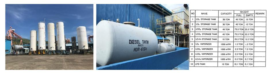
Aboveground storage tanks are spread across the site. Production gas station has oxygen, ethylene, LPG and carbon dioxide storage (left) and capacity has been given in the table (right). The storage tanks for the production gas station and the air receivers at this location have all completed and approved inspection records available. Pre-treatment and paint shop have diesel tanks (mid) which are bunded (good condition) and a carbon dioxide AST.
