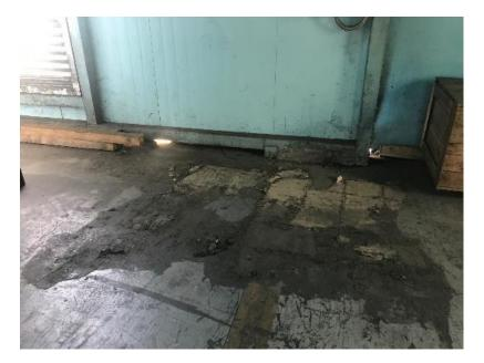
Closed chemical/paint storage has explosion proof lighting, but is insufficiently ventilated (left). Spill was present on the floor (right), which did not spread outside, but the potential is there, due to holes in the walls near the surface level.
