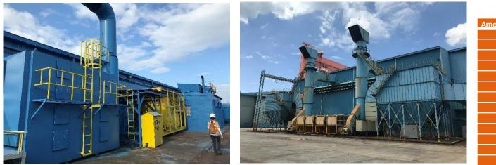
Dust collectors (right) and scrubbers (left) are collecting particles and filtering gases from production processes. Dust collectors are mainly used for blasting and painting processes, whilst the wet scrubbers are used for more intense processes as galvanizing, pre-treatment and alternative paint processes. Waste from the dust collectors are collected in large containers (including filter bag) and transported to the waste storage facility as hazardous waste.
