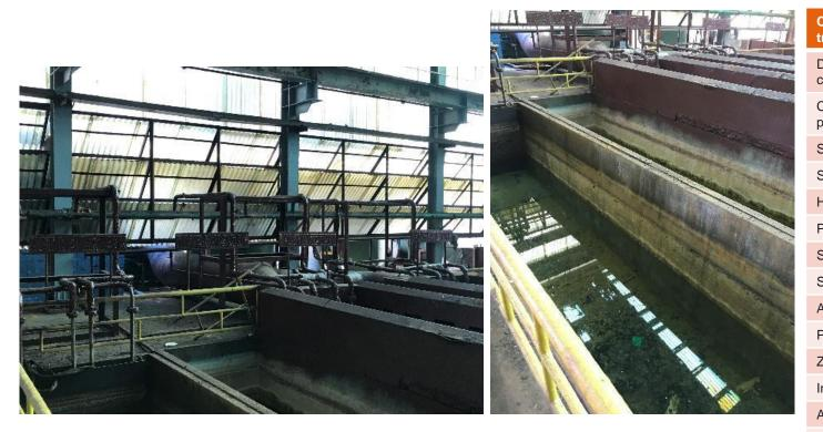
Site personnel informed that contaminated process water from pre-treatment (left and right) and galvanizing is treated in the attached wastewater treatment facility (WT-50, Shinzo) and afterwards is stored in containers and transferred as hazardous waste towards the waste storage area. At the waste storage, the hazardous wastewater is picked-up, transported and disposed of by a contractor. Chemicals used in the pre-treatment and galvanizing process are given in the table to the right.
