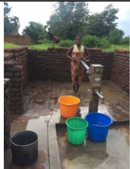
Borehole in Mayambo Village
