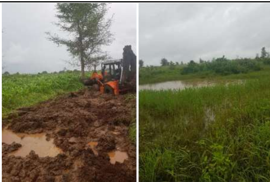
Figure 5.7 Impermeable Clay Layer in Zone One (Source Aurecon, 2018)
