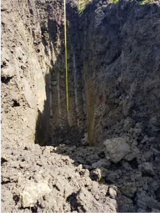
Figure 6: Unstable test pit at Zone 1
