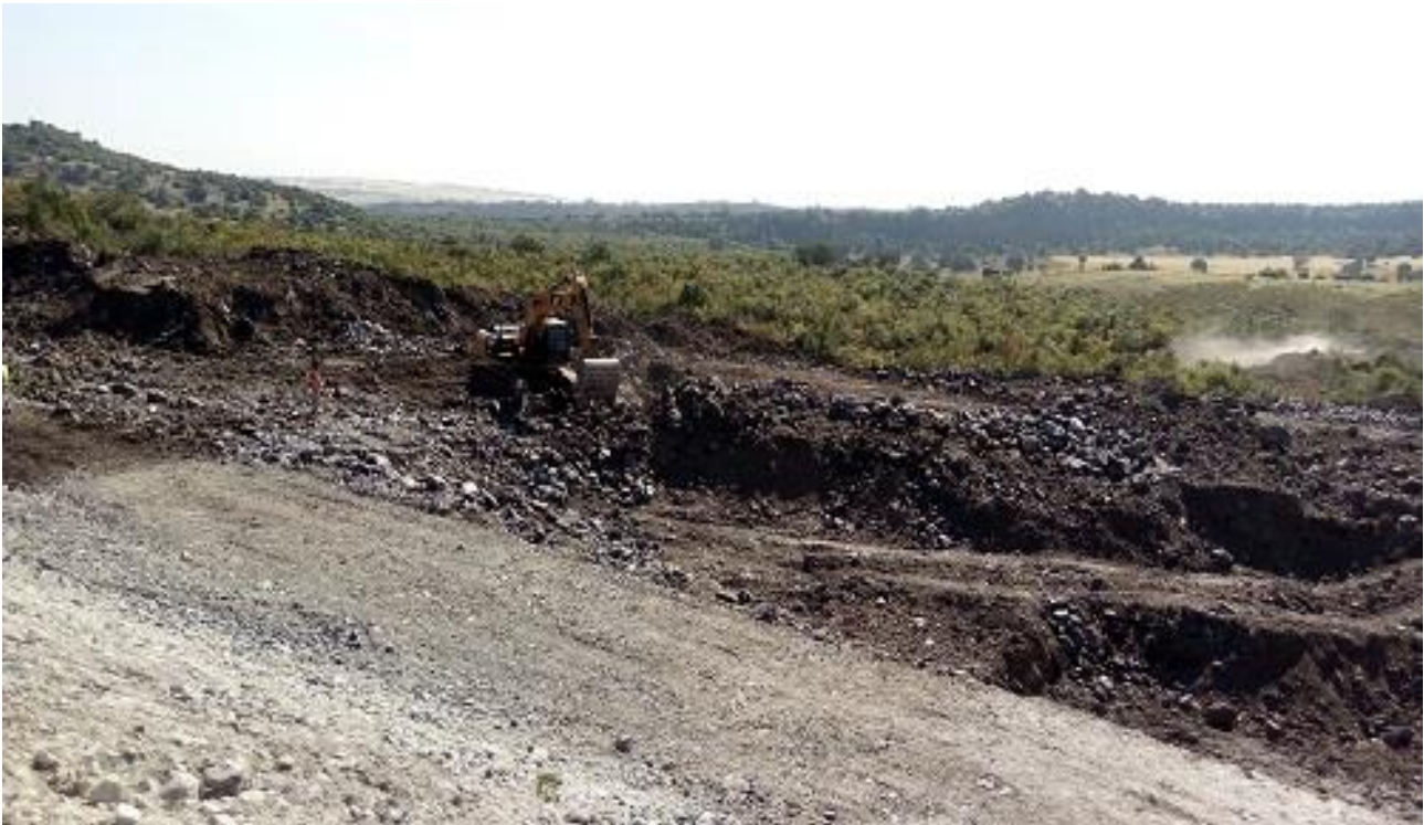
Figure 7-5: Cleared Water Storage Pond Site under Construction Surrounded by Dense Natural Vegetation
