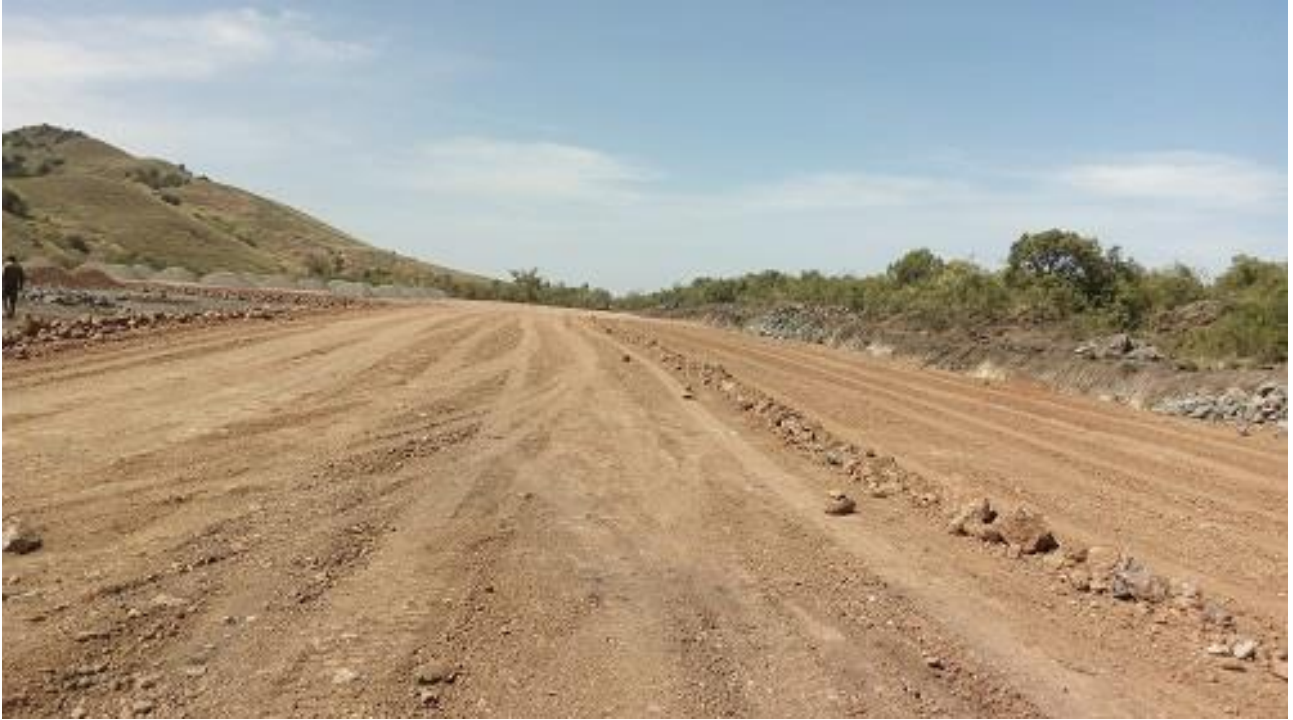
Figure 7-2: Cleared Drill Pad A under Construction
