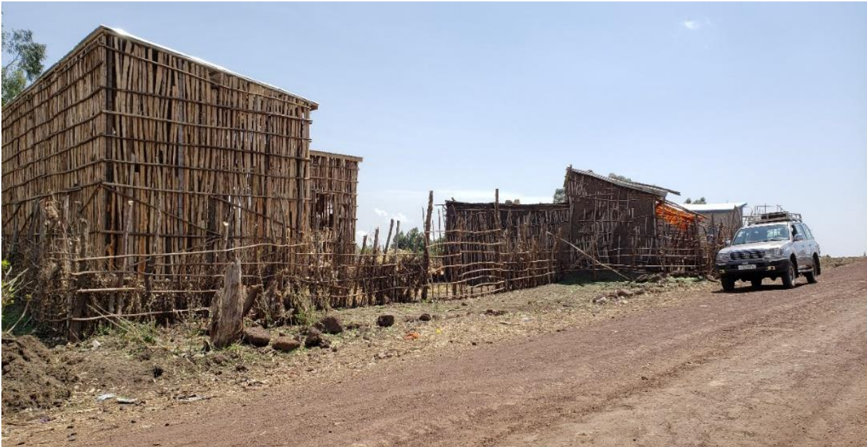
Figure 24: Compensated House (pictured right) and New House being Rebuilt (pictured left) 60
