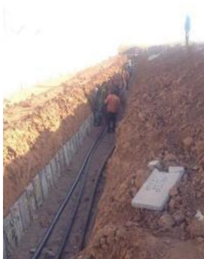
Figure 13 - Example of cable installation work
