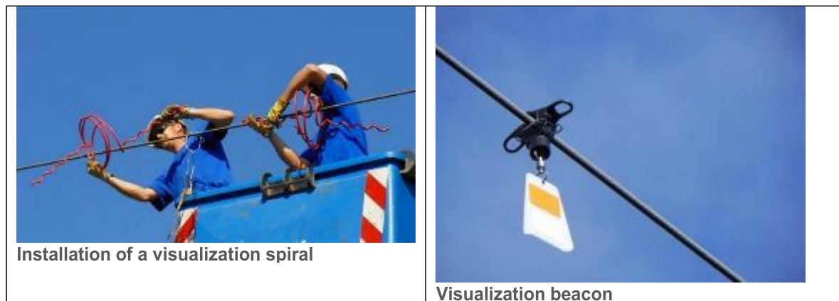
Figure 45 - Example of bird protection devices
