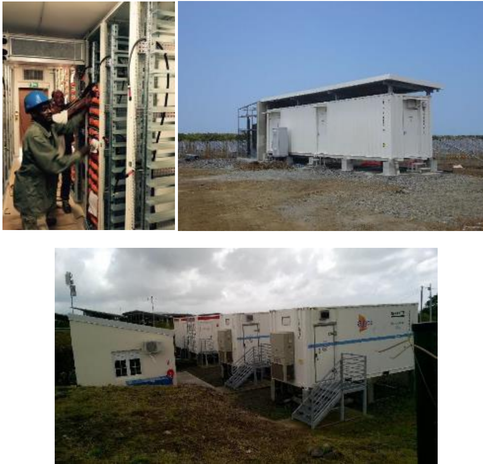
Figure 10- Example of a battery backup system
