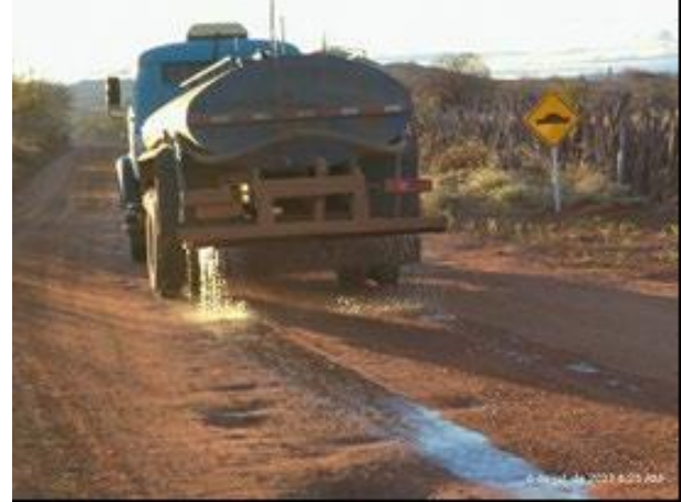
Picture 14 – Road sign installed and water sprinkling on access road.
