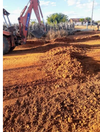
Picture 12 – Bumps built by PNM close to communities and households for speed (safety) and dust control.
