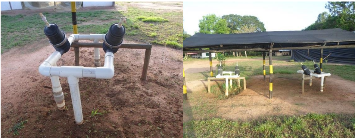
Figure 3.19: Sediment filter for the irrigation system
