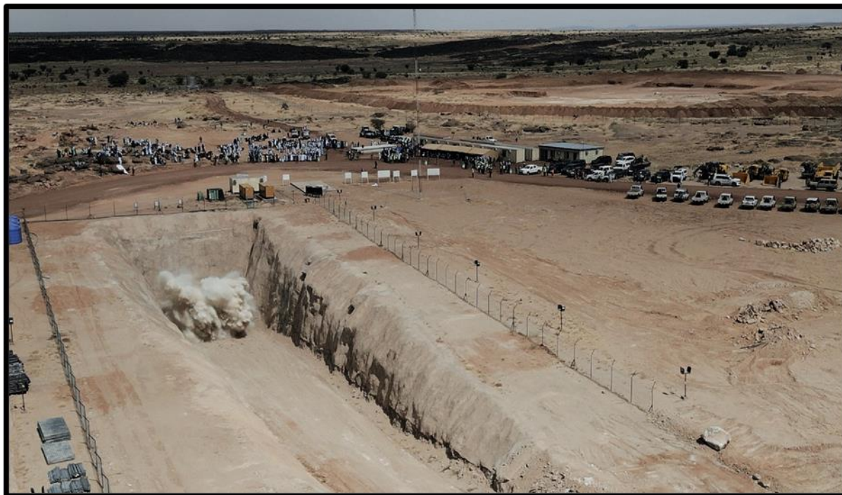
Figure 3-2: Opening blast ceremony, November 5, 2022; underground development begins
