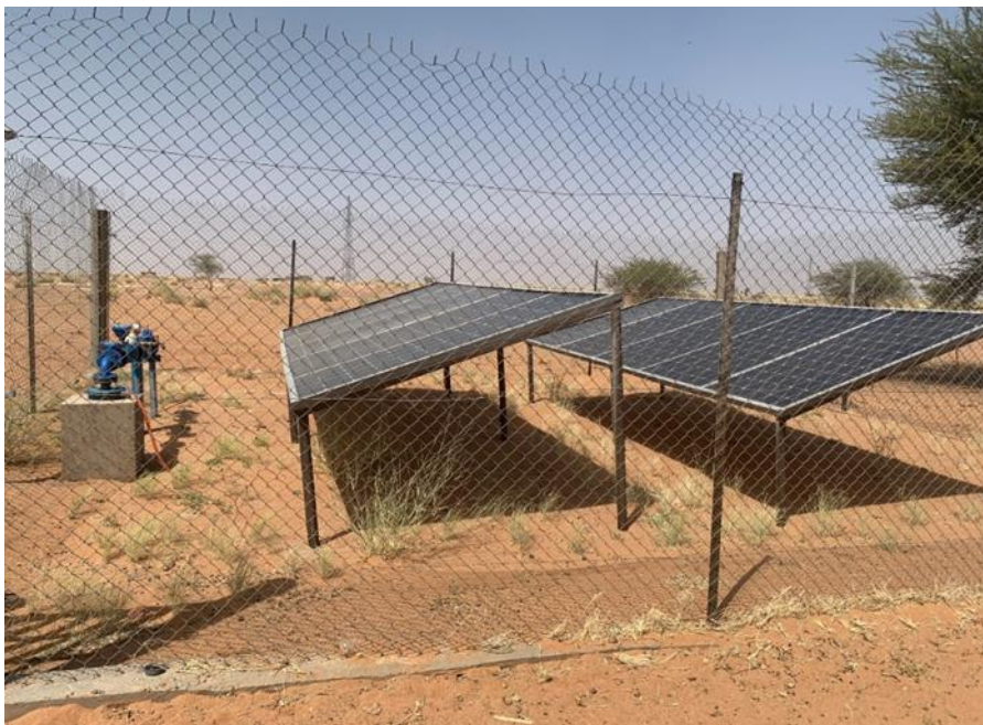
Figure 6-10: A solar-powered water pump near the Dasa Project
