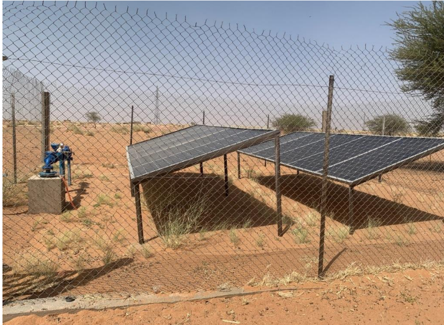
A solar powered water pump near the Dasa Project.
