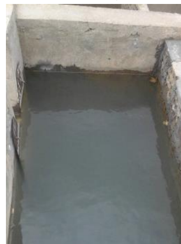
Water storage tank for mountain spring S-11
