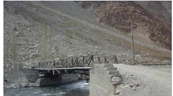
Bridge for vehicles in the Study Area
