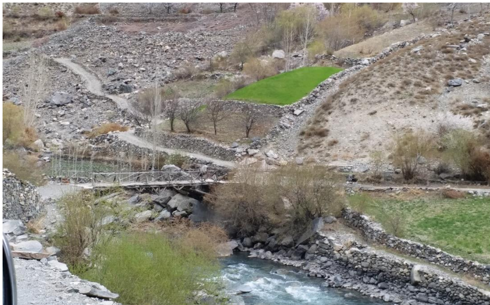
Exhibit 7.18: Access Road near Dam Site
