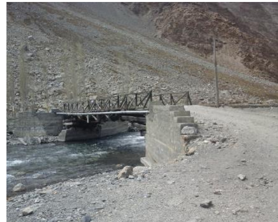
A bridge for vehicles
