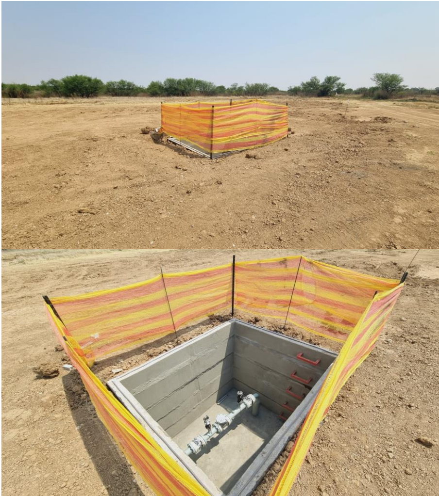
Figure 9: Typical example of a pre-cast well chamber.
