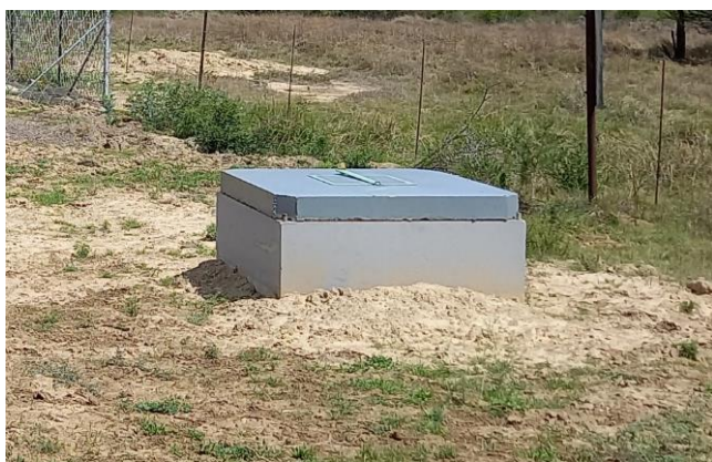
Figure 11: View of an existing low point drain constructed as part of Cluster 1.
