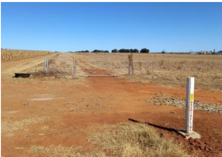
Figure 8: Typical pipeline servitude and pipe marker.
