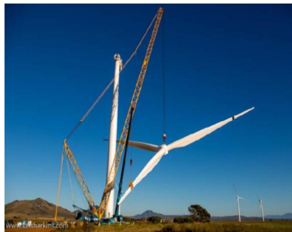
Rotor Lift: crane supporting blade tip until necessary ground clearance is achieved.
