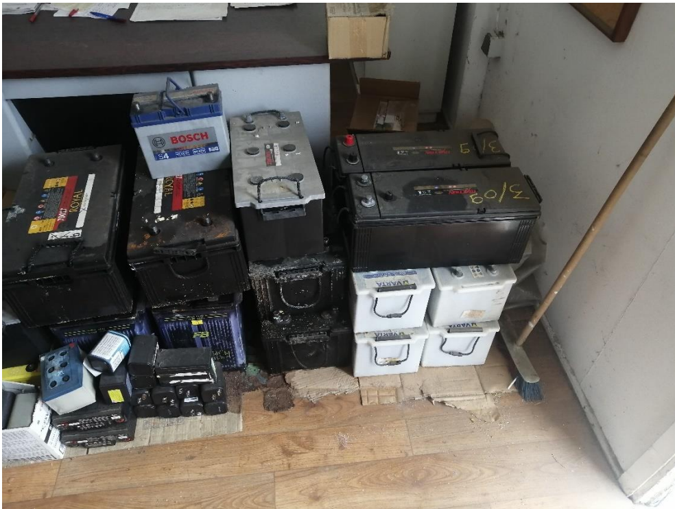
Figure 3.20: Used Batteries Storage Area
