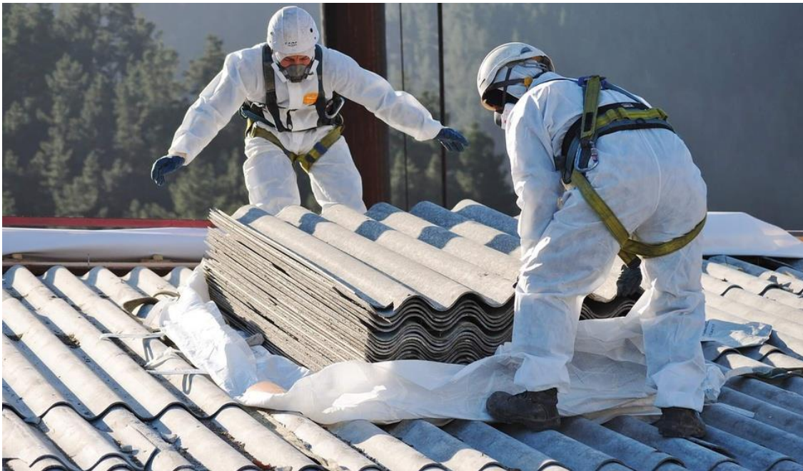
Figure 17.1: ACM removal from similar surface
