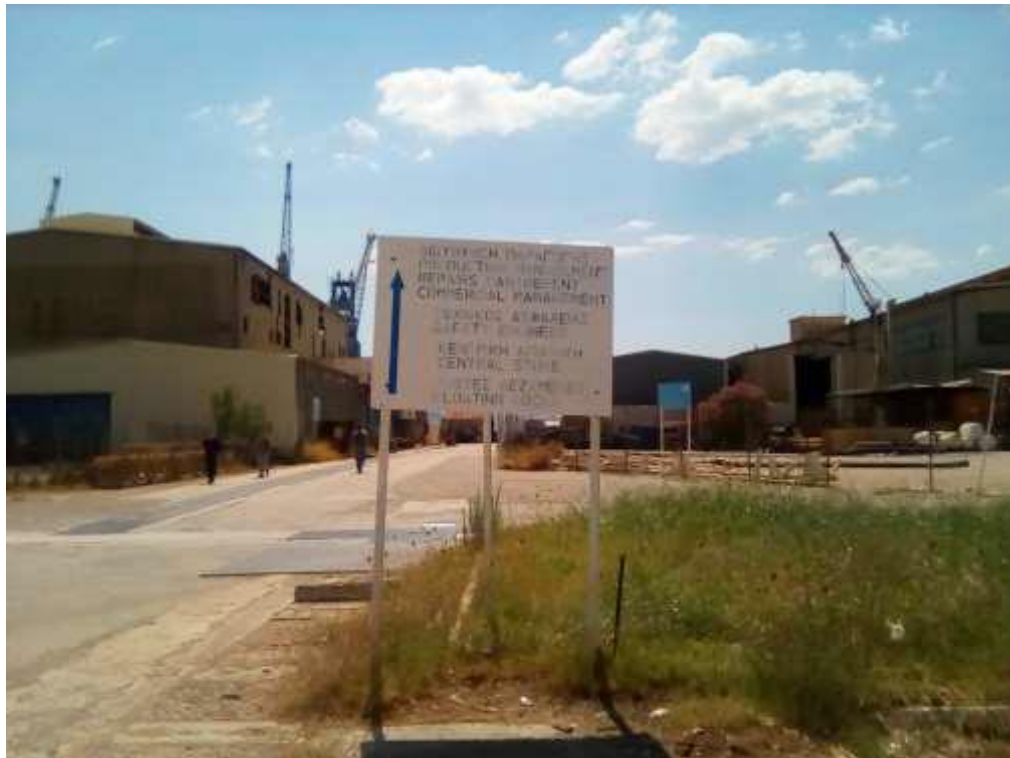
Figure 3.10: Typical Direction Sign not conforming with traffic standards
