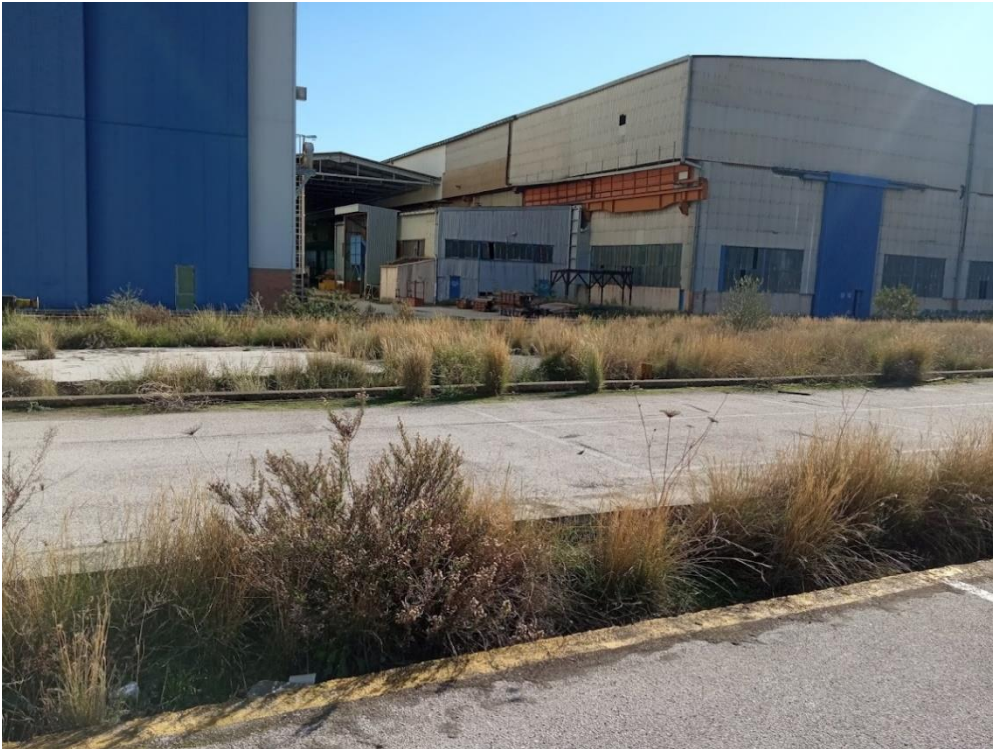
Figure 3.11: Closer view of internal road network
