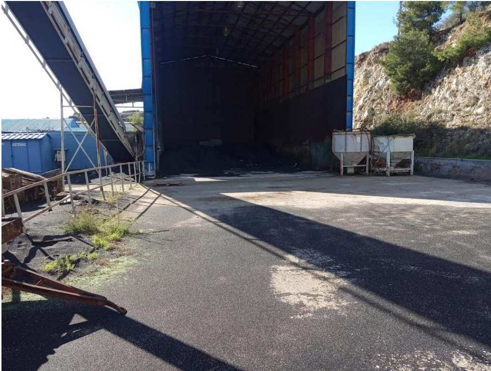
Figure 3.13: Sandblast waste storage Area 1
