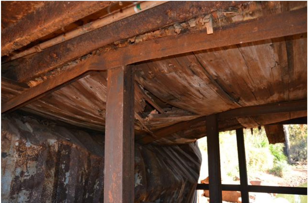
Plate 4.4: The disintegrating underside of bridge 2 (July 2013)
