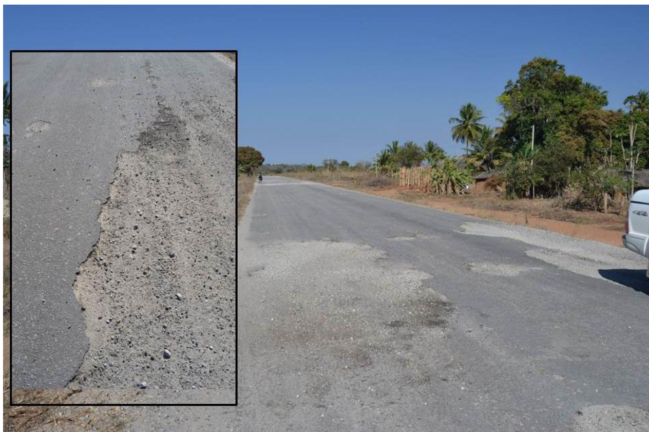
Plate 4.1: The patchy, broken tar for about 15 km west of Montepuez (July 2013)
