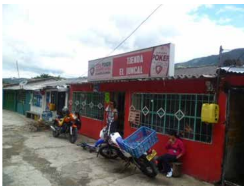
Photograph 5.13 Commercial structure of the infrastructure in place in the El Juncal rural district.
