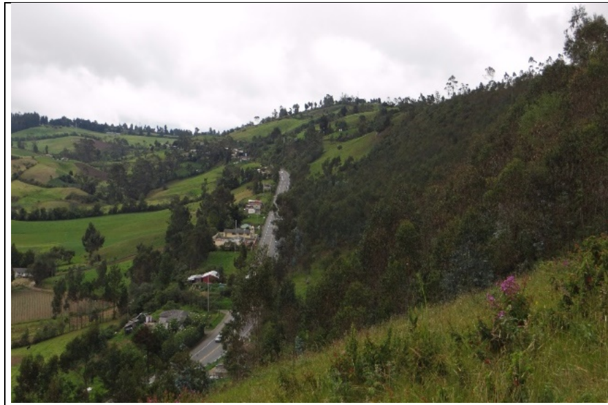
Photograph 2.20 Pan shot of RUMICHACA - PASTO's DUAL CARRIAGE WAY PROJECT, PEDREGAL - CATAMBUCO SPAN, sampling point for FU5. Coordinates (1,132397; - 77,352368)
