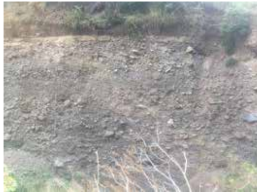
Location X: 957054, Y: 606779. Municipality of Imues
