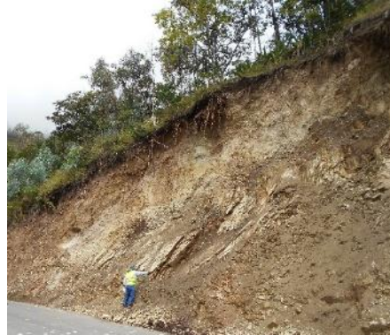
Location X: 955352, Y: 601161. Municipality of Iles Source: GEOCOL CONSULTORES S.A., 2017.
