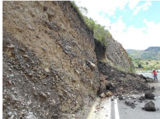
Location X: 955995, Y: 600503. Municipality of Iles Source: GEOCOL CONSULTORES S.A, 2017.
