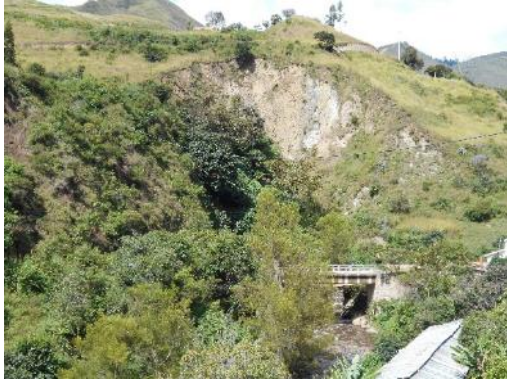
Location X: 954841, Y: 605081. Municipality of Iles Source: GEOCOL CONSULTORES S.A., 2017.
