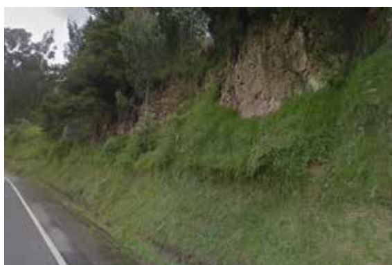
Photography 5-93 Outcrop of Rumichaca Ash Reservoirs (Qdcr).
