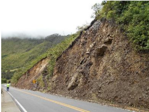
Location X: 955135 Y: 600975. Municipality of Iles Source: GEOCOL CONSULTORES S.A, 2017.
