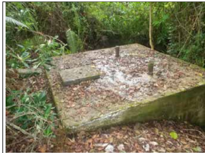
Image 5.3.65 Aqueduct in La Merced, Planar Coordinates, Origin Magna Colombia E 973159.504 N 617968.133 Source (Géminis Consultores Ambientales S.A.S, 2016)
