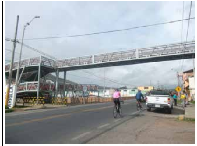
Image 5.3.72 Catambuco pedestrian bridge, Planar Coordinates, Origin Magna Colombia E 976300.783702423 N 620841.410109473 Source (Géminis Consultores Ambientales S.A.S., 2016)
