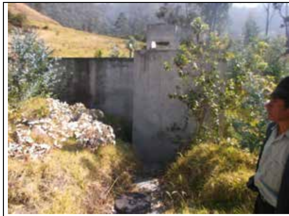
Image 5.3.32 Bolívar Neighborhood Aqueduct, Planar Coordinates Origin Magna Colombia E 965065,774 N 613104,880 Source (Géminis Consultores Ambientales S.A.S, 2016)
