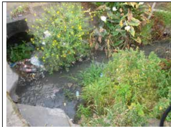
Image 5.3.66 Sewage in San José de Catambuco, Planar Coordinates, Origin Magna Colombia E 976153.309 N 620767.55 Source (Géminis Consultores Ambientales S.A.S, 2016)
