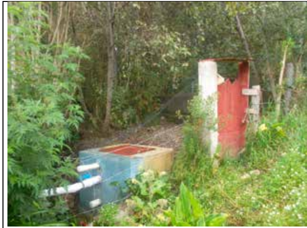
Image 5.3.63 Aqueduct in Taminango - Catambuco, Planar Coordinates, Origin Magna Colombia E 975213.352 N 620121.42
