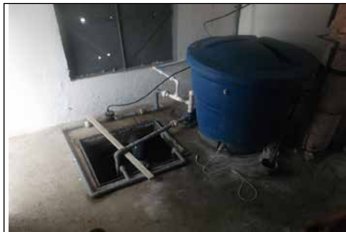
Image 5.3.4 Tangua Nariño Aqueduct - Chlorine plant. Planar Coordinates Origin Magna Colombia E 964290,350685744 N 613194,639896887
