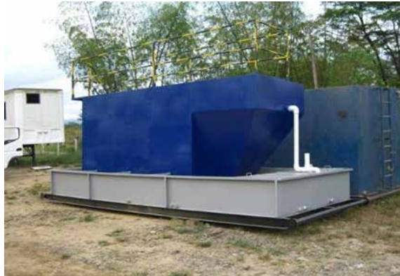
Photograph 7.14 Typical Treatment Plant
