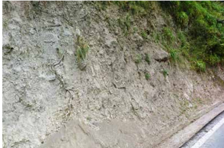
Photography 5.1.4: Pyroclastic deposits, volcanic brecciae in tuffy matrix in the k 3 + 510
