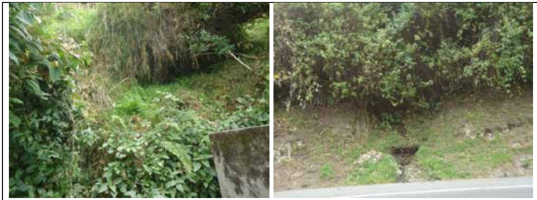
Photography 5.162 Water point PA-M-35 and Water point PA-M-36
