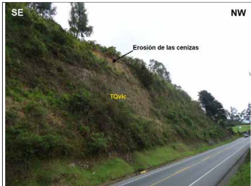
Photography 5.1.29 Talus with erosive processes in the TQvic unit
