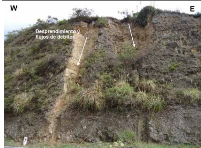
Photography 5.117 Landslide process in the lahars and pyroclasts unit identified in the talus of the current road at K16+220
