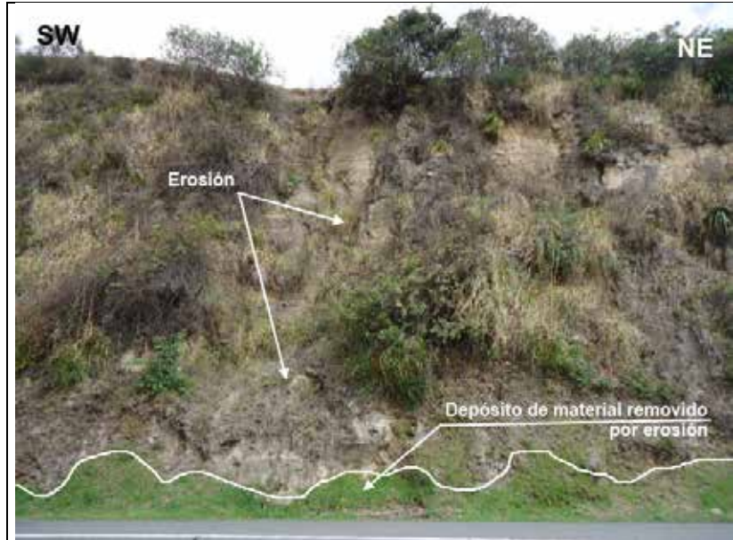
Photography 5.118 Talus on the current road evidencing active erosion processes
