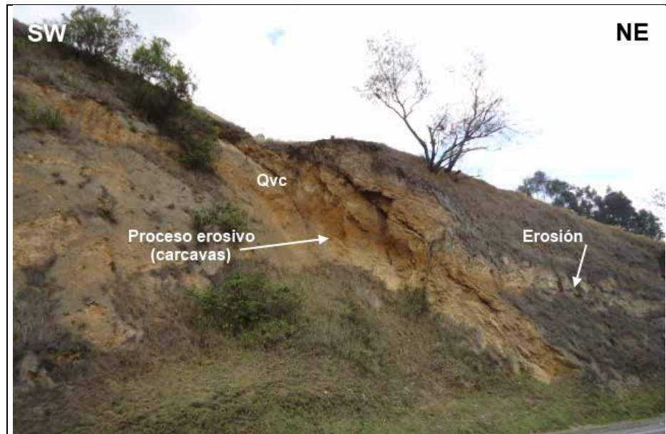
Photography 5.1.36 Talus in the current road presenting gully erosion.
