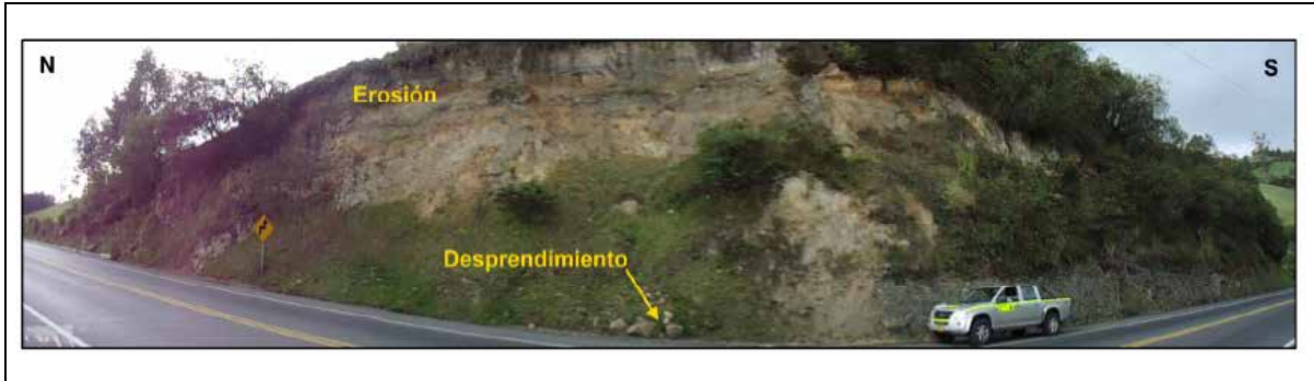
Photography 5.1.30 Talus with landslide processes.
