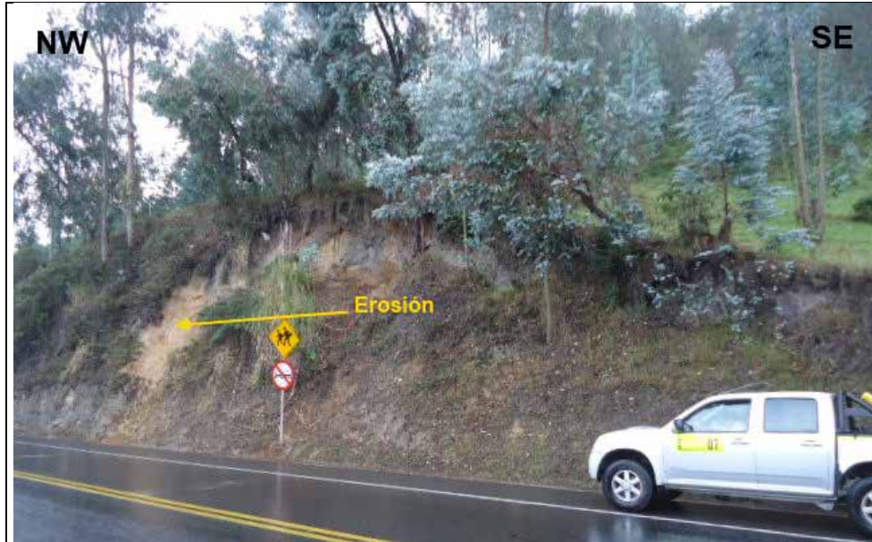
Photography 5.1.32 Talus on the current road with erosive processes
