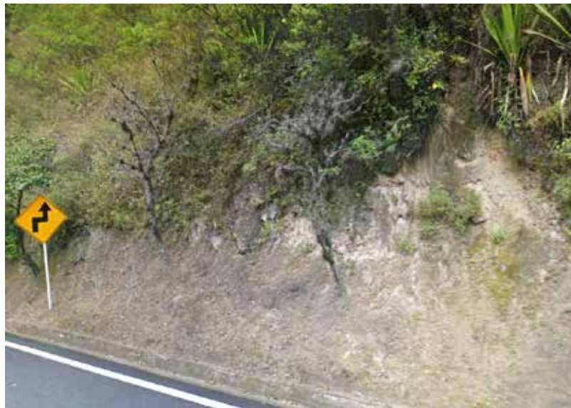
Photography 5.1.4: Pyroclastic deposits, volcanic brecciae in tuffy matrix in the k 3 + 510
