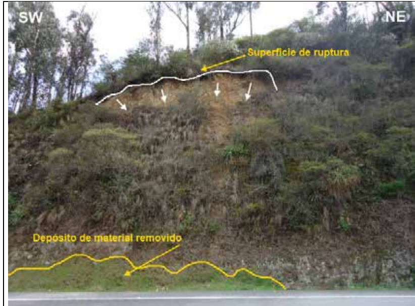
Photography 5.116 Scar from a landslide process, the removed material deposit due to the process may be observed in the lower part.
