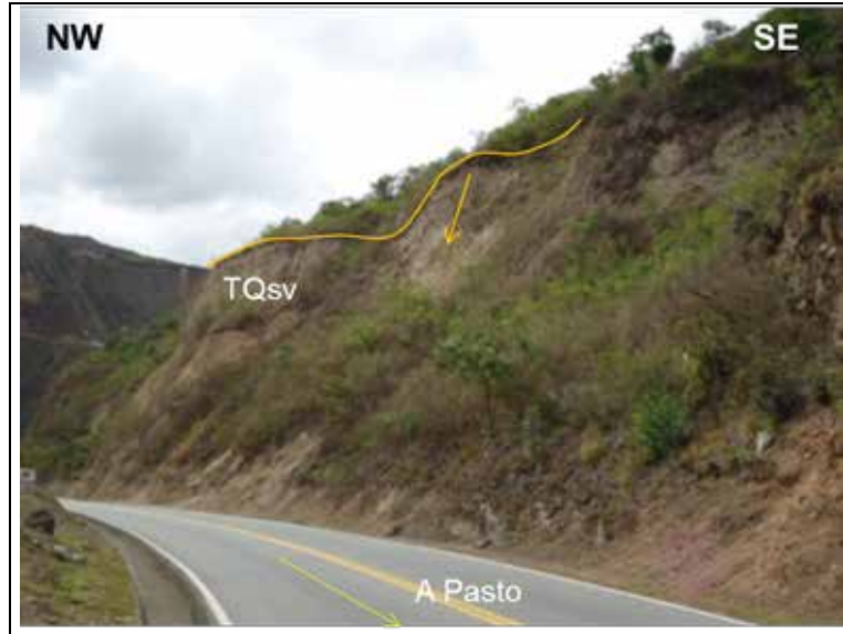
Photography 5.1.27 Surface and slight erosion with presence of furrows in the TQsv unit in K3+100
