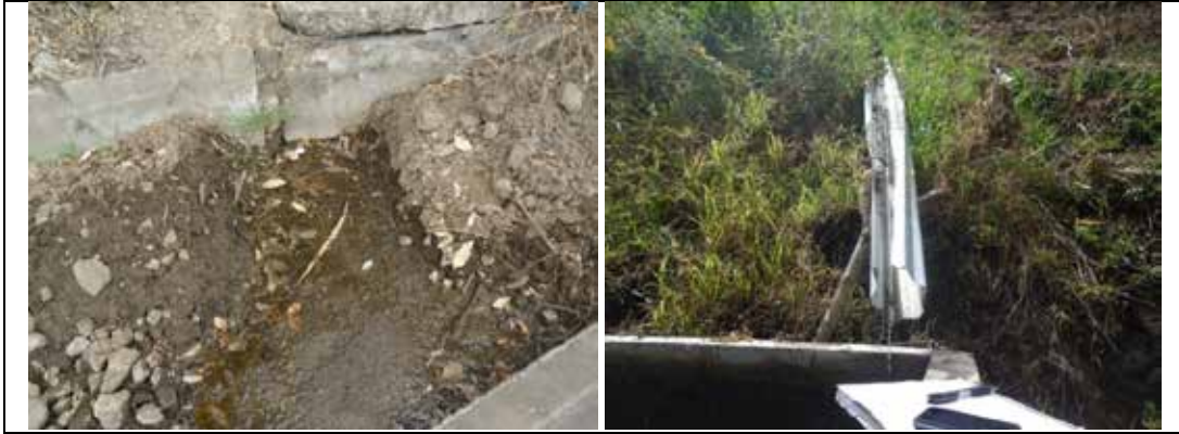
Photography 5.161 Water point PA-M-33 and Water point PA-M-34
