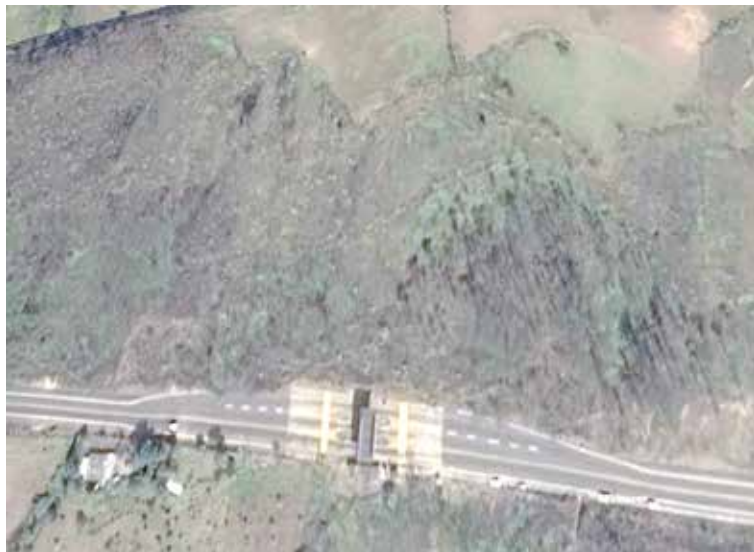
Photography 5.1.8: Colluvial deposit generated by landslide in the toll area.
