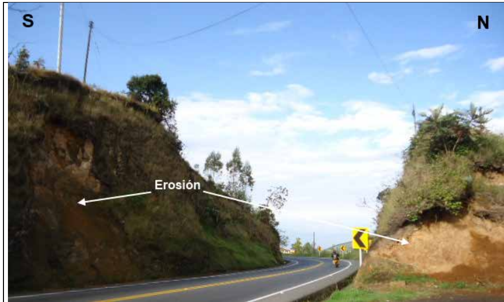
Photography 5.1.34 Current road talus with erosive processes.
