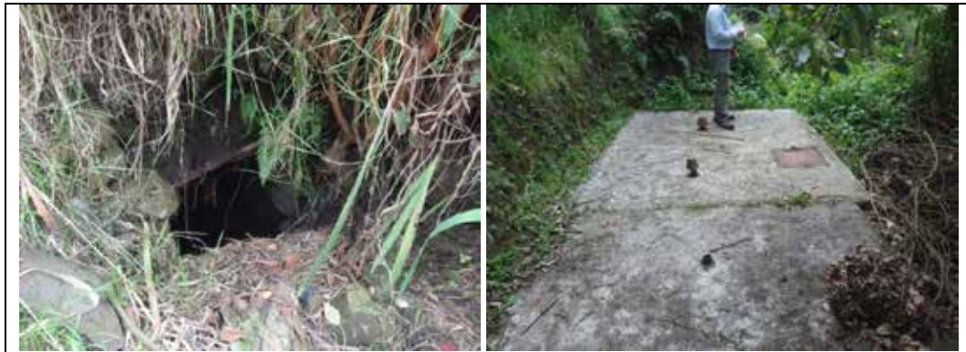
Photography 5.165 Water point PA-M-41 and Water point PA-M-42
