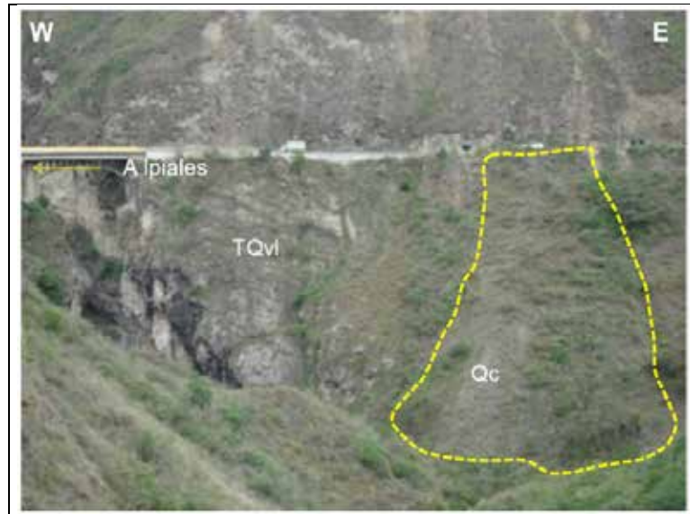
Photography 5.1.14 Colluvial deposit (Qc) between the abscissas K3 + 060 and K3 + 070 Source (INGETEC, 2016)
