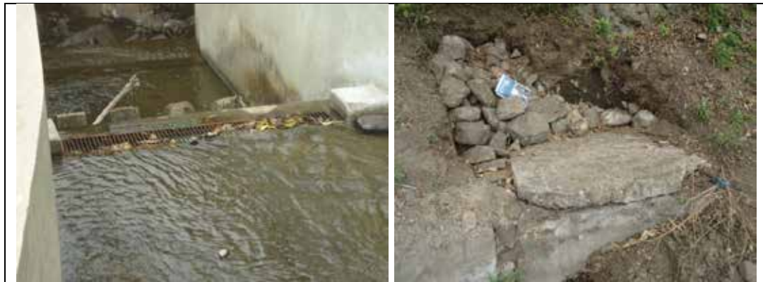
Photography 5.1.60 Water point PA-M-31 and Water point PA-M-32
