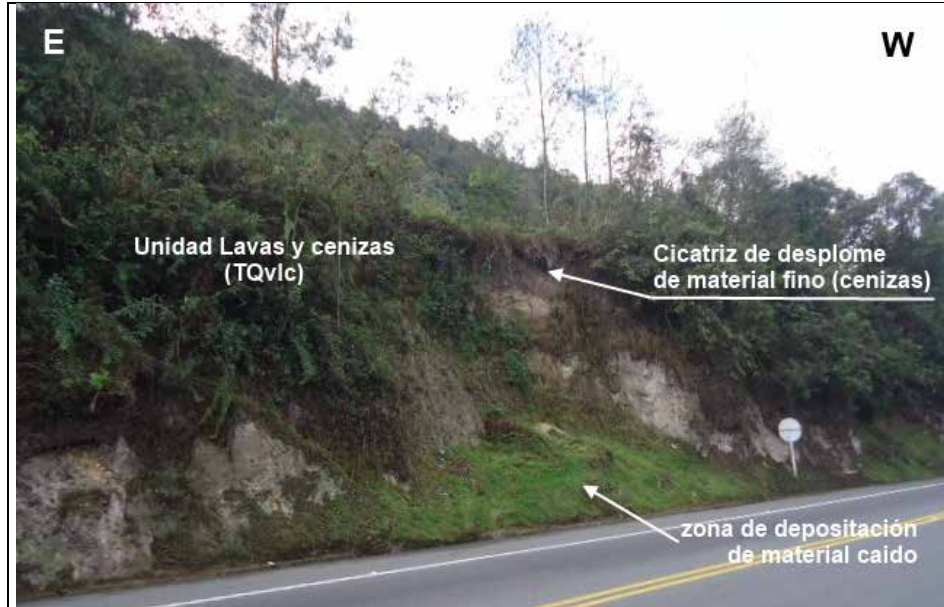
Photography 5.1.33 Talus of the current road with collapse of fine material scar from the TQv/c unit.
