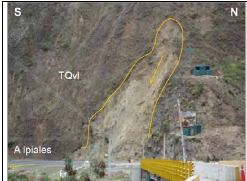
Photography 5.1.24 Detritus flow in TQvl at the height of K2+800
