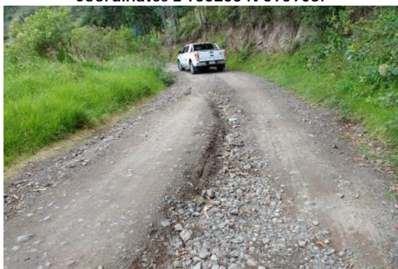
Photograph 3.47 KP3+707. Road section with damage to surface due to lack of runoff water management.
