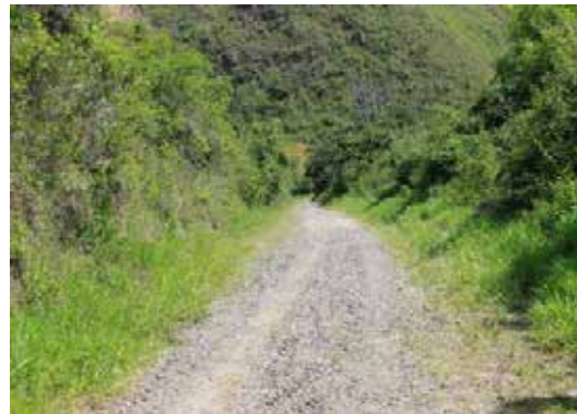
Photograph 3.50 KP2+080. Road section, granular material, roadway 3.0 m wide. Coordinates E 954701 N 602639.
