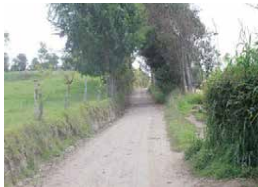
Photograph 3.33 KP8+687. Road section, granular material, roadway 3.50 m wide. Coordinates E 951300 N 595176.
