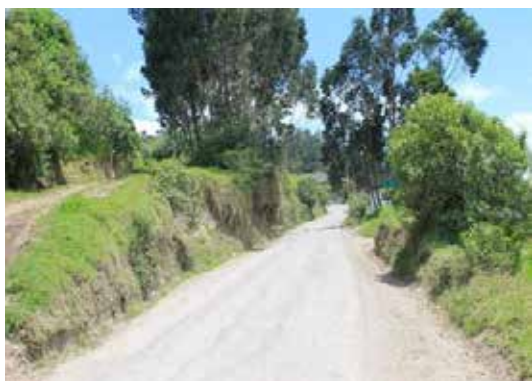
Photograph 3.30 KP0+715. Road section, granular material, roadway 4.50 m wide. Coordinates E 947856 N 592436.
