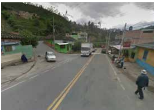
Photograph 3.26 KP2+113. Flexible pavement road section, roadway 6.00 m wide. Coordinates E 947970 N 591508.
