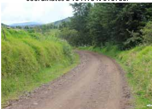
Photograph 3.39 KP10+911. Road section, granular material, roadway 4.00 m wide. Coordinates E 954173 N 598736.
