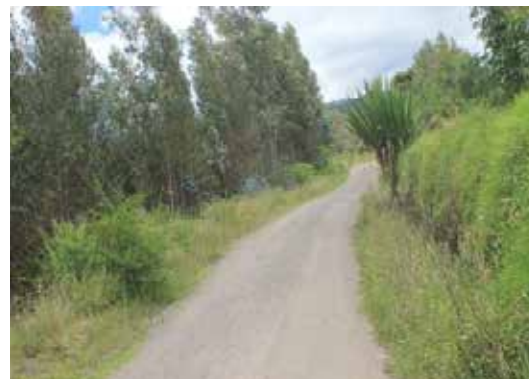
Photograph 3.66 KP1+897. Road section, granular material, roadway 3.0 m wide. Coordinates E 948470 N 591426.
