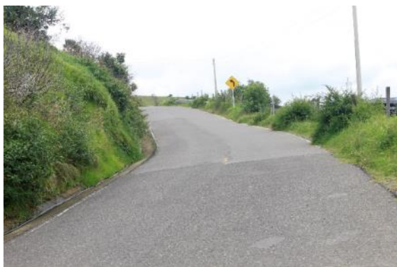
Photograph 3.20 KP7+732. Change in road characteristics. Flexible pavement, with a roadway up to 6.0 m wide, lacks road markings. Coordinates E 952902 N 601812.
