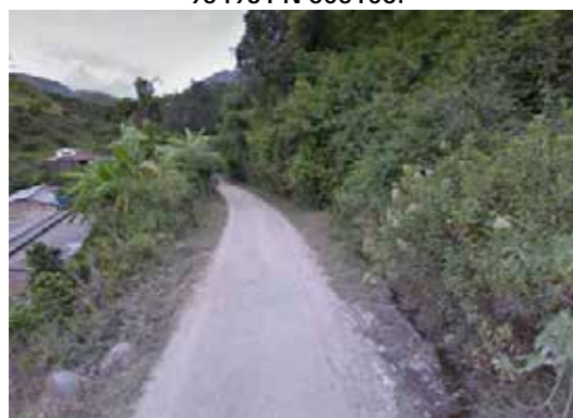
Photograph 3.54 KP0+635. Road section, granular material, roadway 3.00 m wide. Coordinates E 954931 N 605106.
