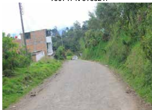
Photograph 3.40 KP15+831. Road section, granular material, roadway 4.00 m wide. Coordinates E 950747 N 598821.
