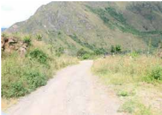
Photograph 3.51 KP4+293. Road section, granular material, roadway 3.5 m wide. Coordinates E 954914 N 603811.
