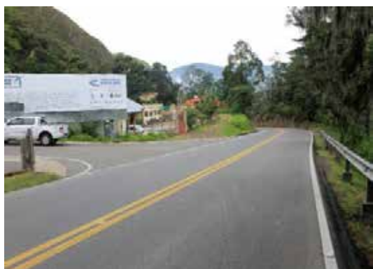
Photograph 3.20 KP7+732. Change in road characteristics. Flexible pavement, with a roadway up to 6.0 m wide, lacks road markings. Coordinates E 952902 N 601812.
