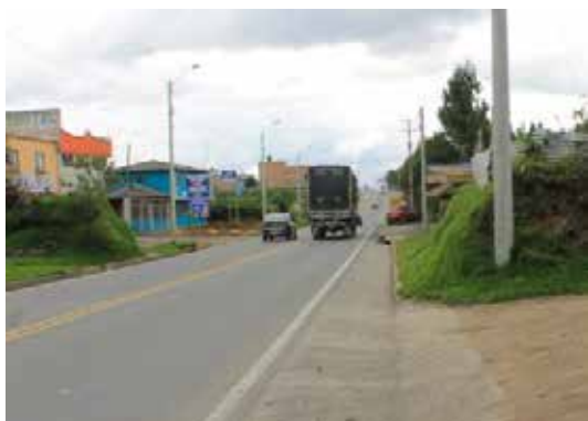
Photograph 3.3 KP8+197. Flexible pavement road section, roadway 7.30 m wide.
