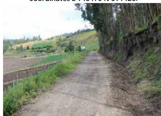
Photograph 3.66 KP1+897. Road section, granular material, roadway 3.0 m wide. Coordinates E 948470 N 591426.
