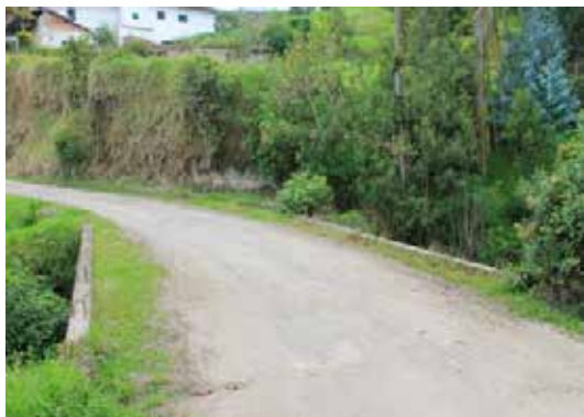
Photograph 3.65 KP1+711. Road section, granular material, roadway 3.0 m wide. Coordinates E 948408 N 591596.
