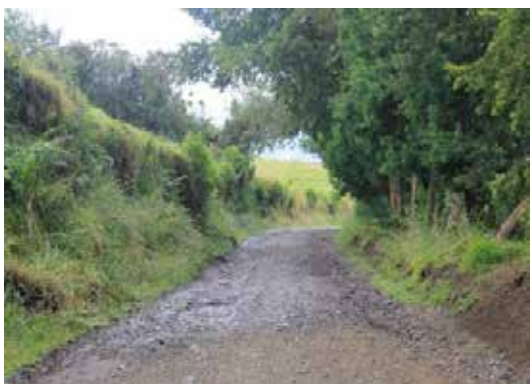
Photograph 3.39 KP10+911. Road section, granular material, roadway 4.00 m wide. Coordinates E 954173 N 598736.
