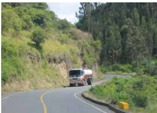
Photograph 3.26 KP2+113. Flexible pavement road section, roadway 6.00 m wide. Coordinates E 947970 N 591508.
