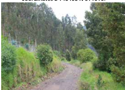
Photograph 3.65 KP1+711. Road section, granular material, roadway 3.0 m wide. Coordinates E 948408 N 591596.
