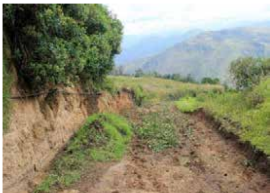
Photograph 3.81 KP0+683. Road section with slope instabilities. Coordinates E 954883 N 601307.
