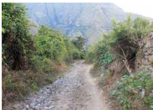
Photograph 3.59 KP2+147. Road section, granular material, roadway 3.5 m wide. Coordinates E 954626 N 603780.
