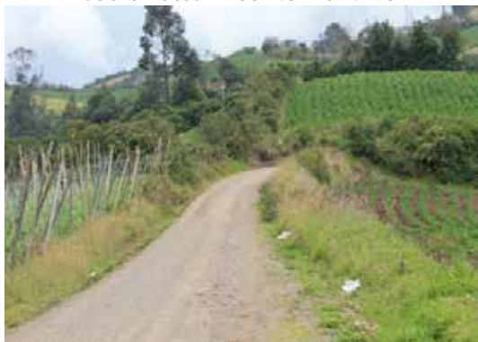
Photograph 3.32 KP5+638. Road section, granular material, roadway 3.50 m wide. Coordinates E 950140 N 594145.
