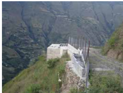
Picture 2.10 Collection Water Pipe at the Arcoiris Condominium (Pilcuan). Coordinates (West Zone Magna Sirgas) E: 954060 N: 604342
