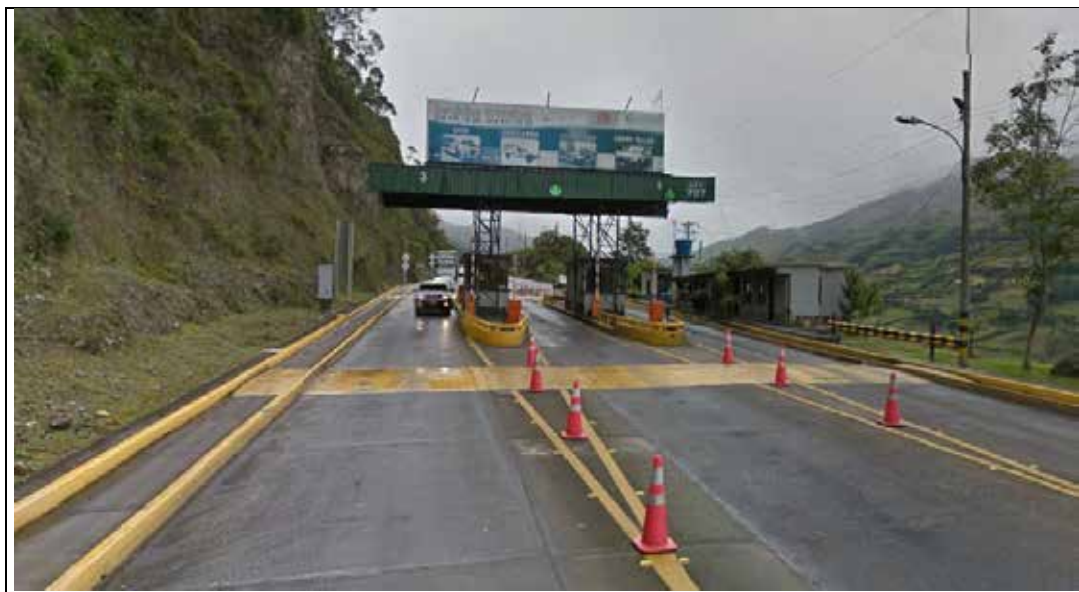
Photograph 3.3 PR49 + 0580 Current El Placer Toll
