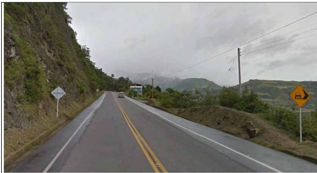
Photograph 3.2 PR48 + 0100 existing road
