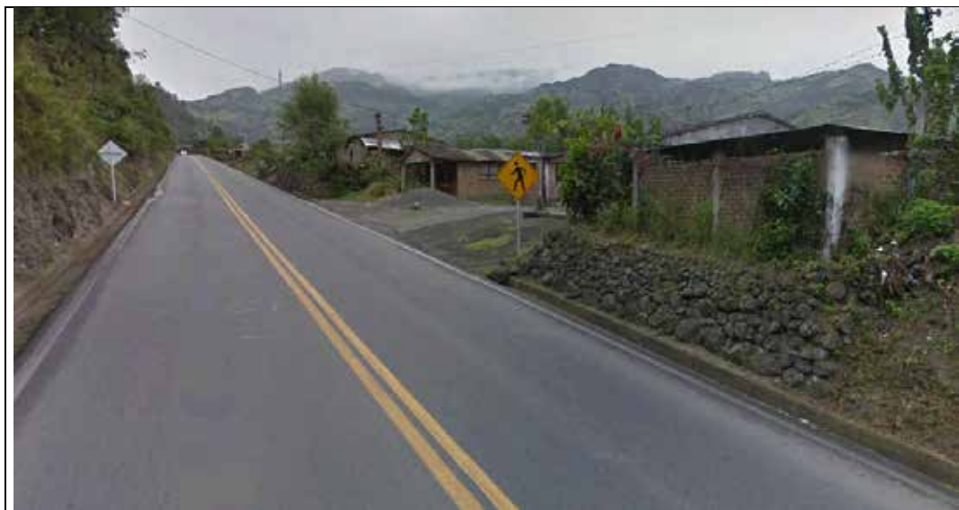
Photograph 3.1 PR48 + 0100 existing road
