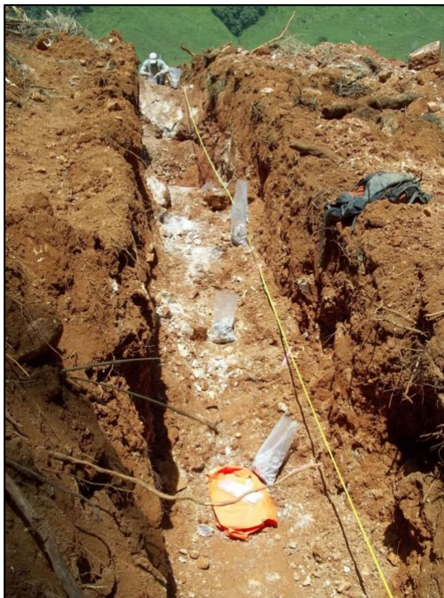
Illustration 2.2-14. T39 trench east of Mining Concession 5969.
