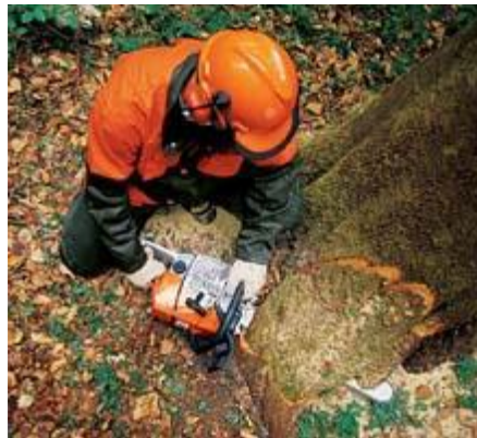
Illustration 8-29. Cut in wedge to direct the fall of the tree. Source: Universidad del Tolima, 2011.
