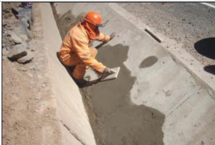
Illustration 8-13. Ditch covered with concrete Source: Guide for routine maintenance of unpaved roads, 2013.
