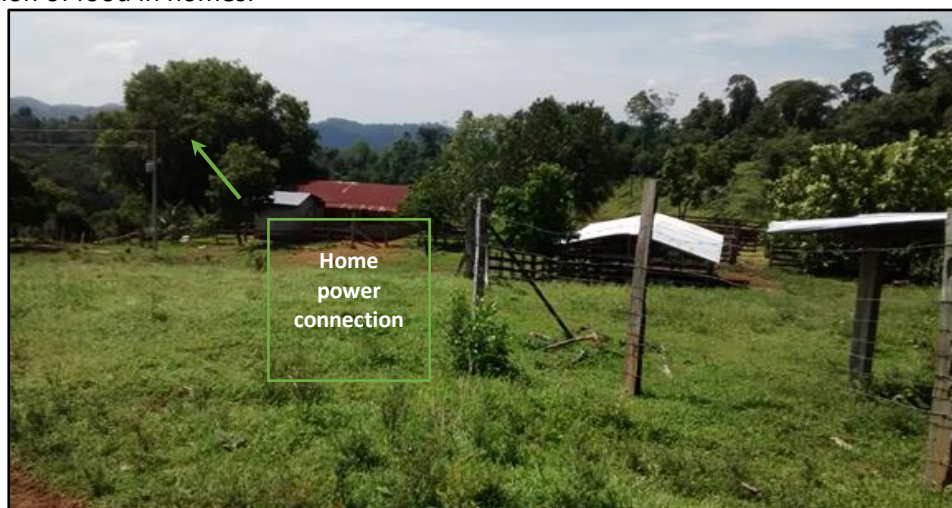
Illustration 4.3-29. Dwelling with AIDL AIDP household electricity connection. Source INGEX, 2015
