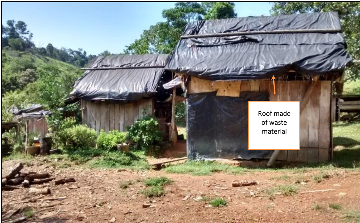
Illustration 4.3-24. Composite dwelling roof waste material, AIDL.
