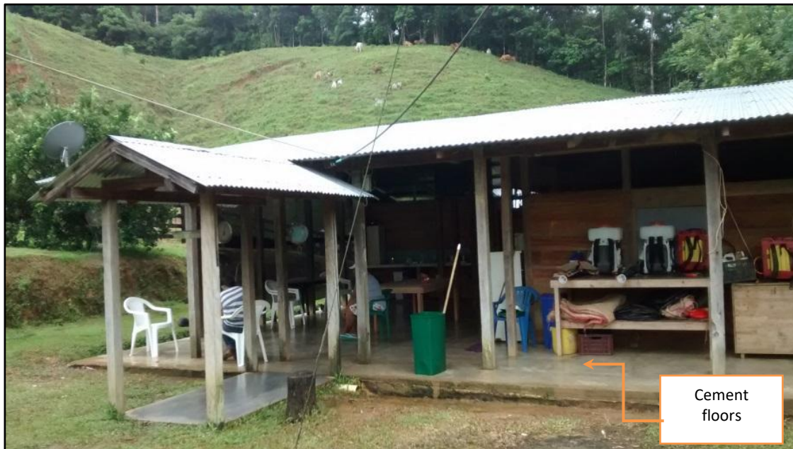
Illustration 4.3-26. Housing with cement floors. Source INGEX, 2015
