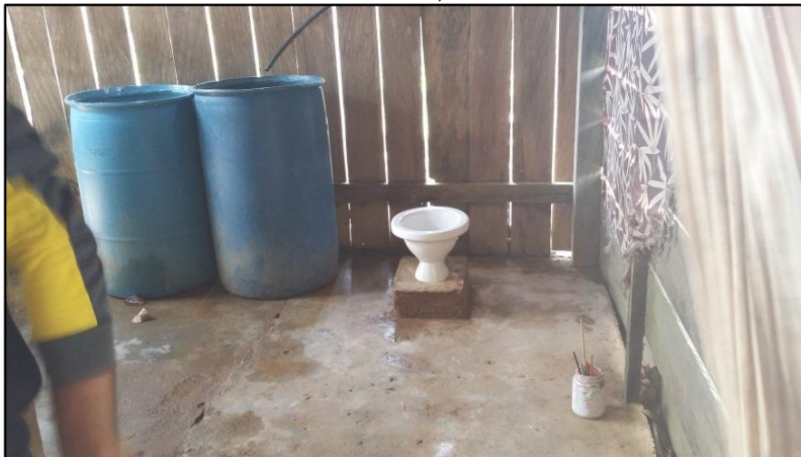
Illustration 4.3-36. Internal part of the sanitary units of the dwellings, in the AIDL AIDP.
