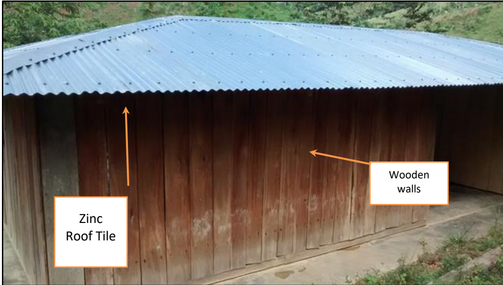
Illustration 4.3-25. Composite housing roof material zinc roof tile and wooden walls, AIDL. Source INGEX, 2015
