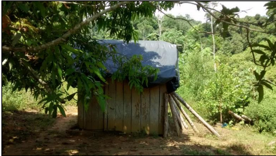
Illustration 4.3-35. External part of the sanitary units in the AIDL AIDP.
