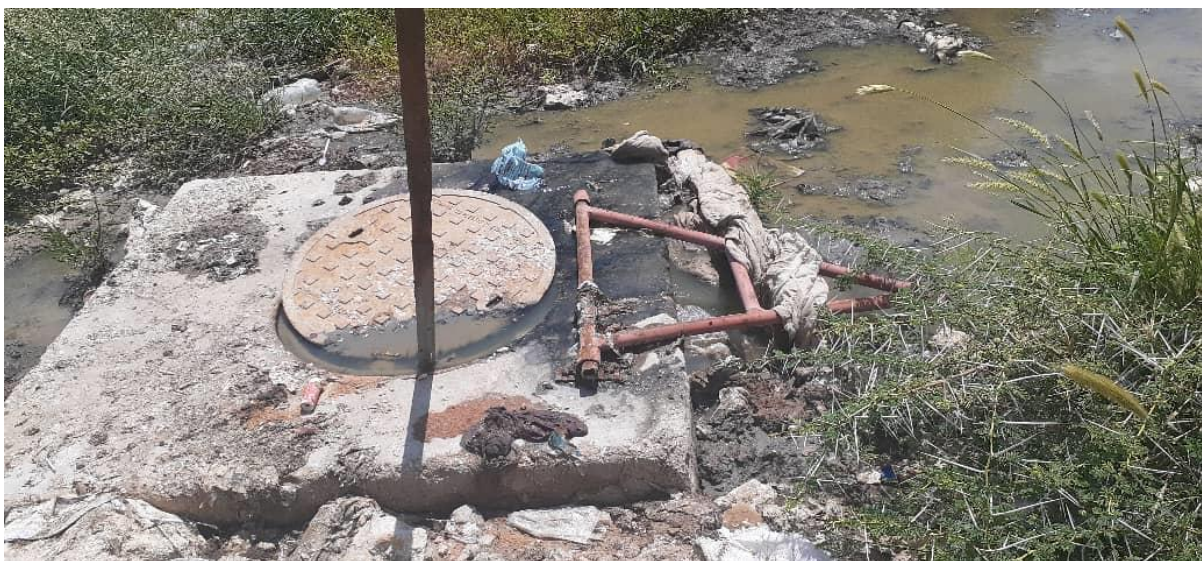
Photo 2: Overflowing sewage system in Usakos
