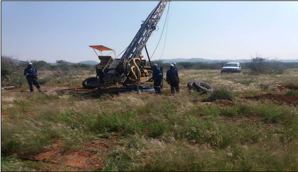
Figure 5 - Photo of a drill site, showing minimum disturbance of the environment
