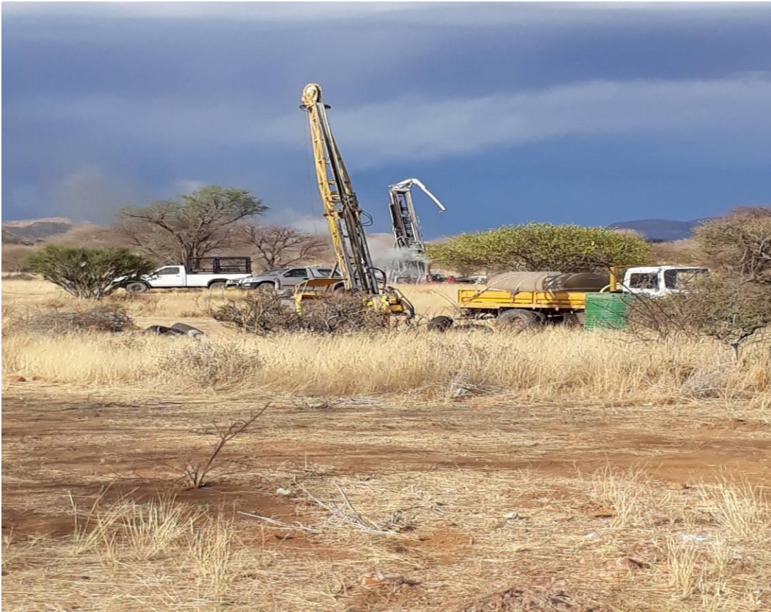
Figure 3 - Photo (DLE) - One diamond Rig & RC rig drilling adjacent to each other at Rubicon
