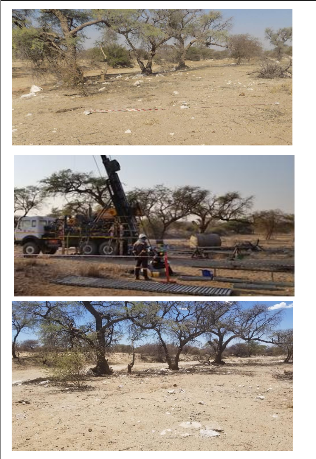
Figure 3 - Photo (DLE); prepared site (top), During drilling (middle), Cleaned up site after drilling (bottom)
