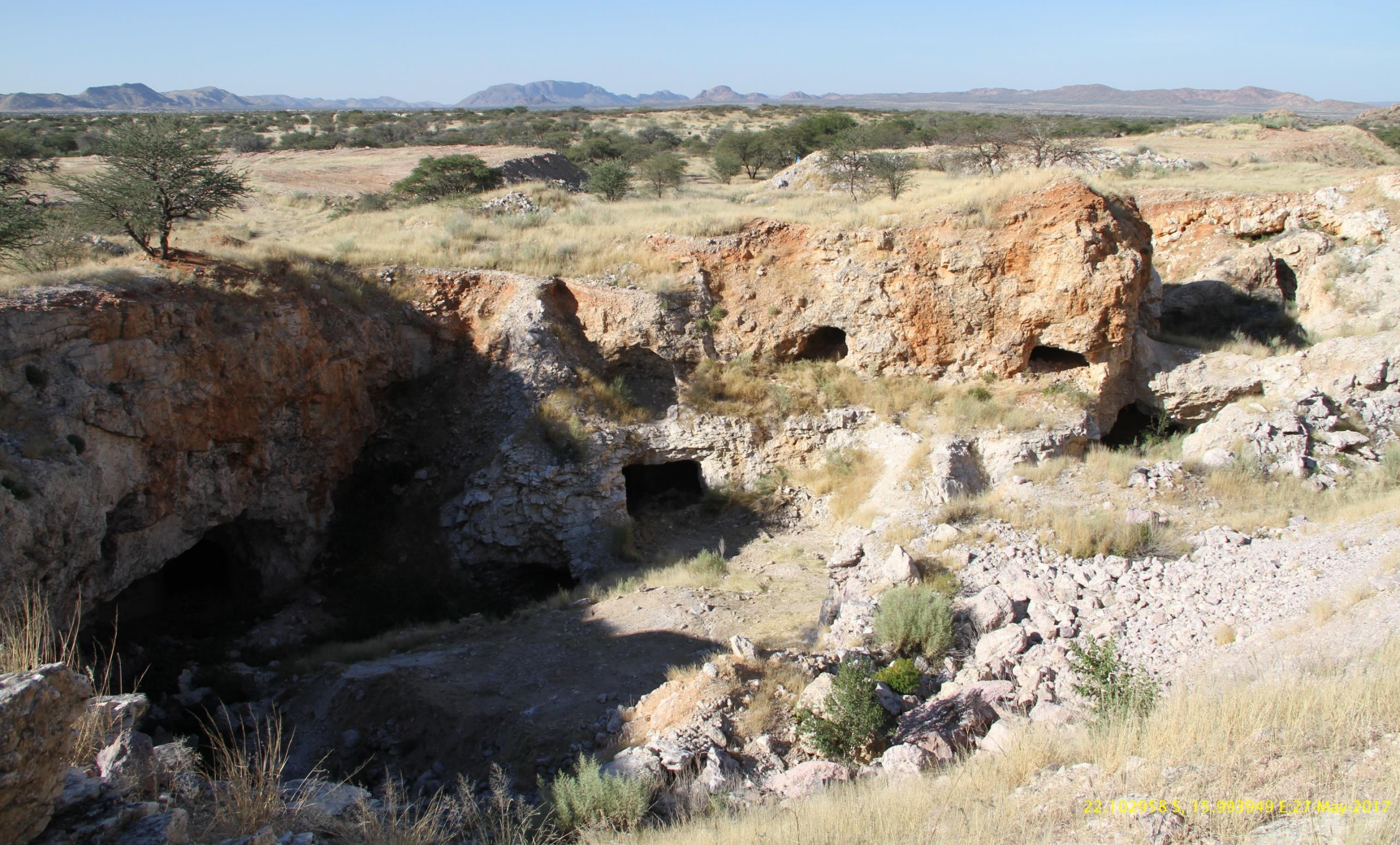
Plate 1.1: Example of the poor state of environment around the Rubicon old mine area showing historical abandoned unstable excavations and shafts that will be subject to extensive remediation, mining and final rehabilitation (RBS Geotagged Image Series, 2017).
