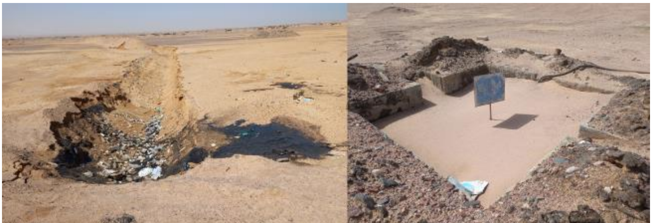
Figure 6-1 - Residual Infrastructure from Oil & Gas Exploration & Extraction
