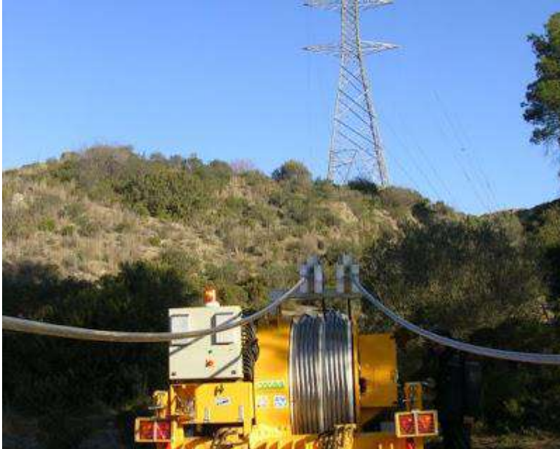
Illustration 6: VIEW OF CONDUCTOR LAYING PROCESS BETWEEN MACHINE AND TOWER.
