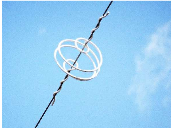
Figure 6.7-1 Spiral Type Bird Flight Deterrent
