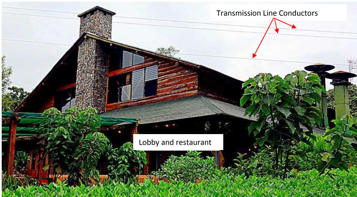
Figure 3: Transmission line crossing Santa Leticia Hotel
