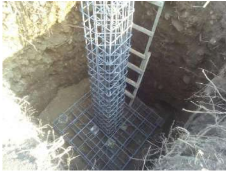
Illustration 1: Foundation of a leg of a tower
