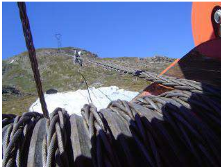
Illustration 5: VIEW OF THE CABLE GUIDE OR PILOT CABLE LAUNCHING PROCESS BETWEEN THE MACHINE AND TOWER.
