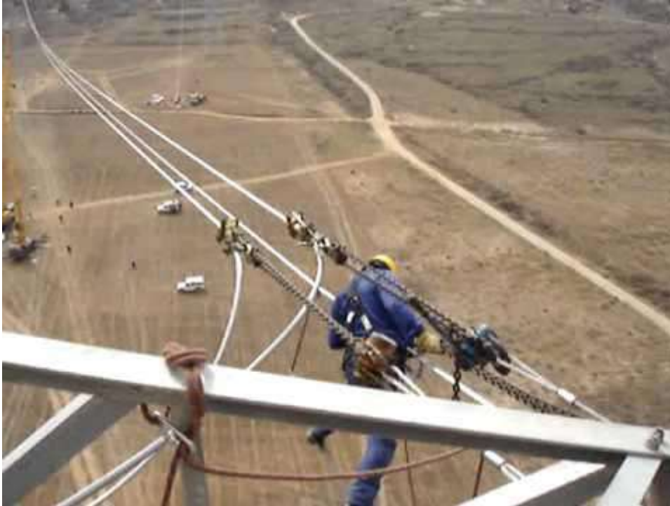
Illustration 10: Technical personnel performing individual cables tensioning in a tower.
