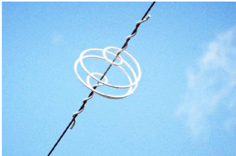
Figura 40. Bird-saving devices Spiral type used to prevent birds from colliding with high voltage cables.
