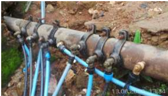
Guma Valley Water Utility Pipe Connection
