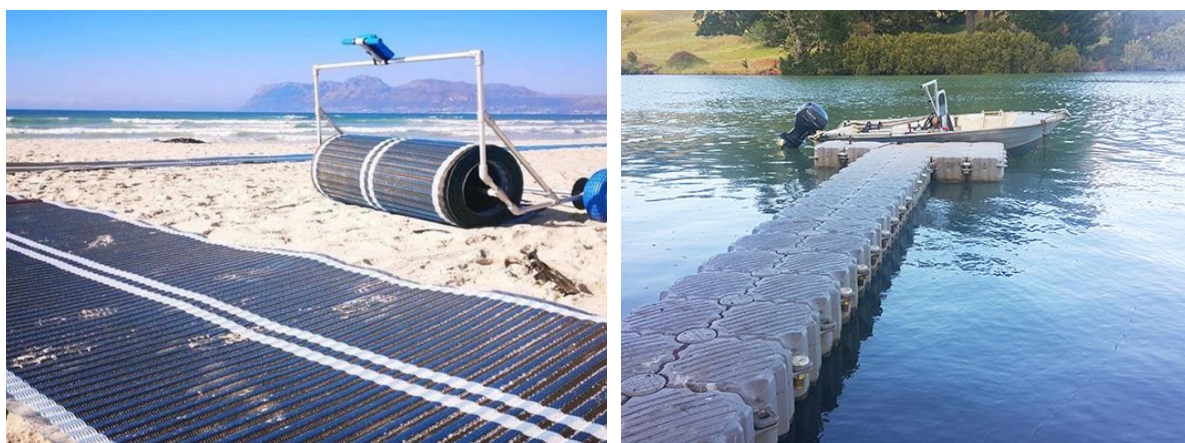
Figure 3: Example of a roll-up ramp (left) and floating jetty (right)
