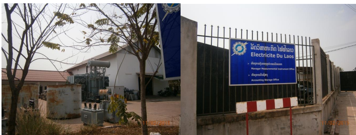
Figure 3-2: EDL Warehouse for Replaced Electrical Equipment
