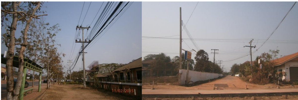
Figure 3-1: Existing 22 kV Distribution ROW
