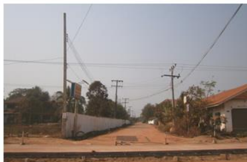
Typical Poles for 22kV Distribution Line
