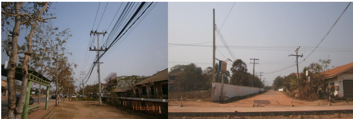
Figure 3-1: Existing 22 kV Distribution ROW
