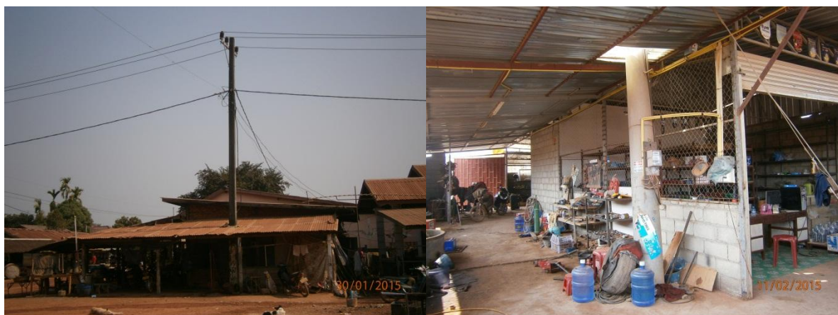
Figure 3-4: Encroachment of Household Structures to Distribution ROW
