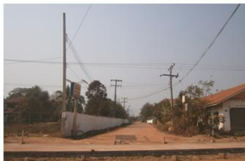
Typical Poles for 22kV Distribution Line
