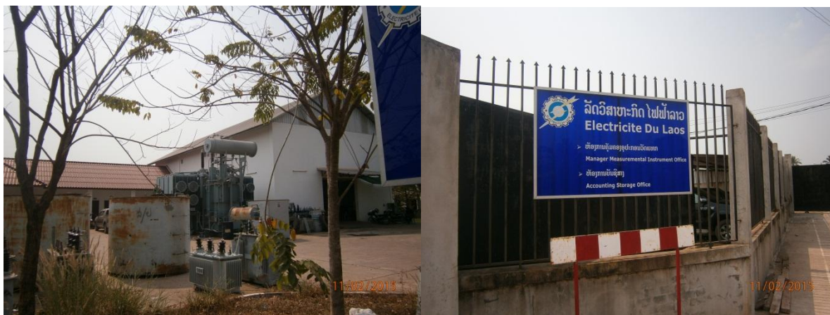
Figure 3-2: EDL Warehouse for Replaced Electrical Equipment
