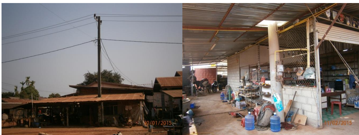
Figure 5: Encroachment of Household Structures to Distribution ROW
