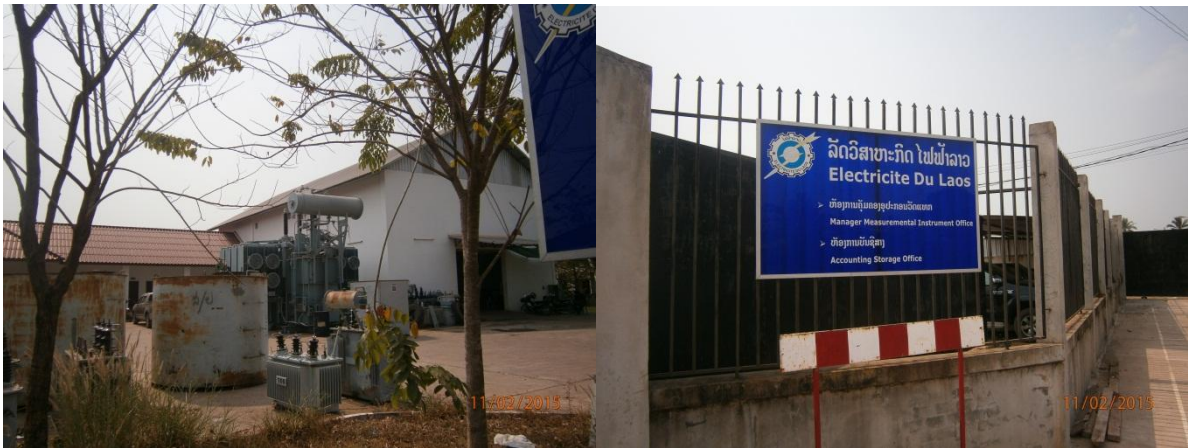
Figure 2: EDL Warehouse for Replaced Electrical Equipment
