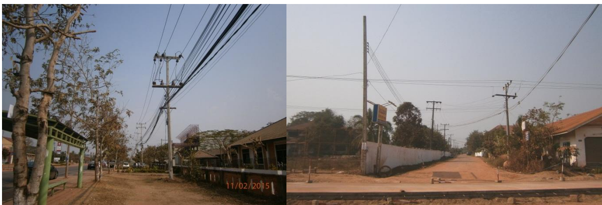
Figure 1: Existing 22 kV Distribution ROW
