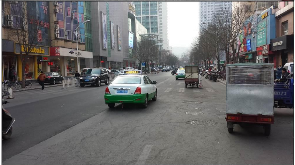
The new road (Wu Yun Bridge - Xinhua Road) 01
