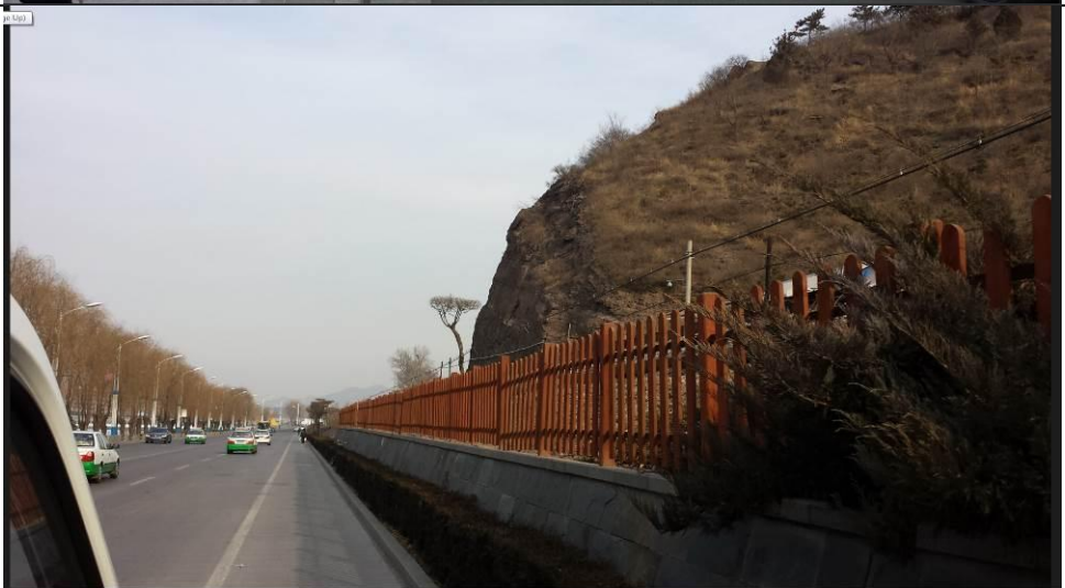
The East Ring Road (Anyuan Temple Bridge South Bridge -)
