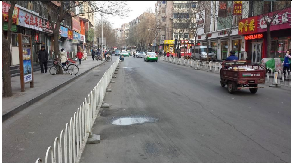
The new road (Wu Yun Bridge - Xinhua Road) 03
