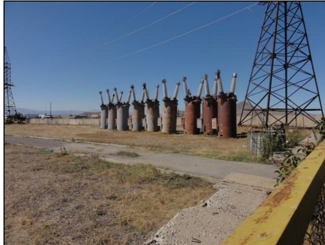
Photo 5-3: Storage of old circuit breakers at s/s Ashnak
