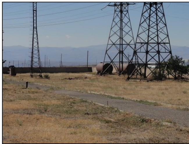
Photo 5-1: Oil storage site at s/s Ashnak
