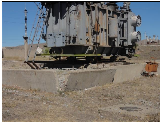
Photo 3-1: Bunds around a transformer are broken at s/s Ashnak
