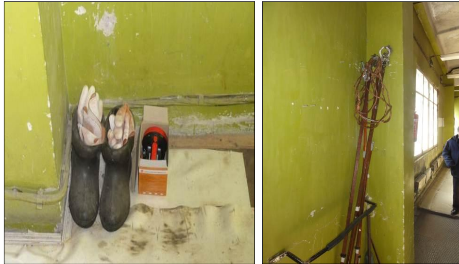
Photo 4-4: Safety equipment and tools for working under high voltage at s/s Ashnak
