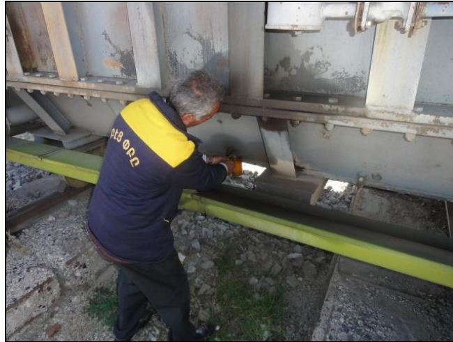
Photo 4-6: Taking of oil samples from transformer at s/s Ashnak
