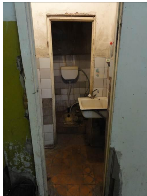
Photo 4-5: The only toilet at s/s Ashnak
