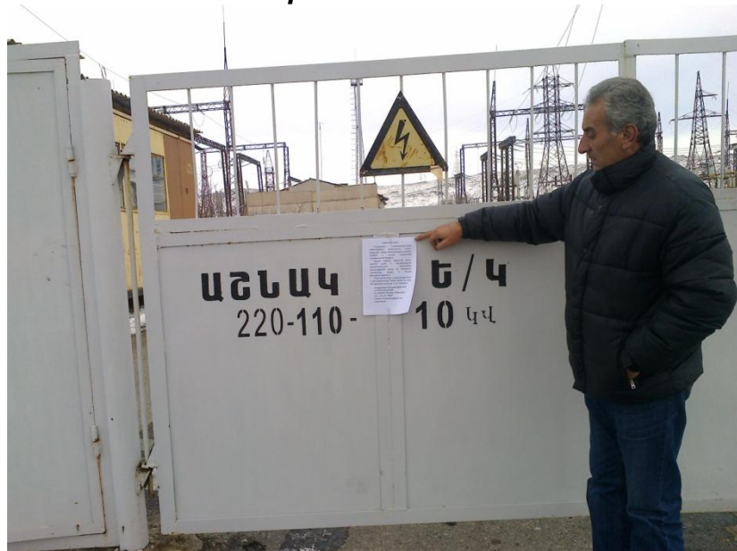
Photo: Notifications placed at Ashnak substation
