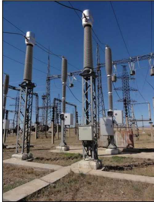
Photo 3-3: SF 6 circuit breakers installed in 2010 at s/s Ashnak
