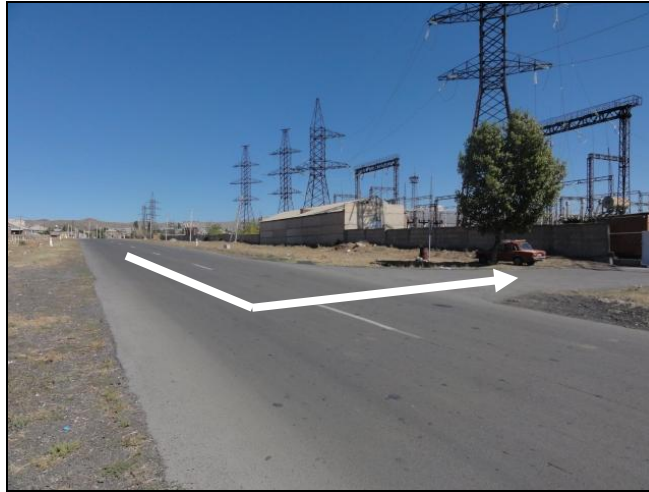
Photo 3-4: Wide access to substation site at s/s Ashnak
