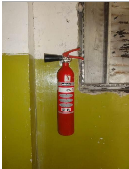
Photo 4-3: Fire extinguisher (powder) inside control building at s/s Ashnak
