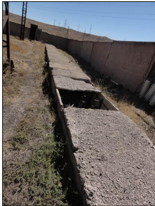
Photo 4-1: Badly maintained cable ducts at s/s Ashnak
