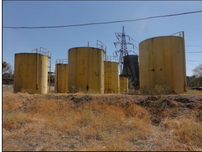
Photo 5-1: Oil storage site at s/s YTPC
