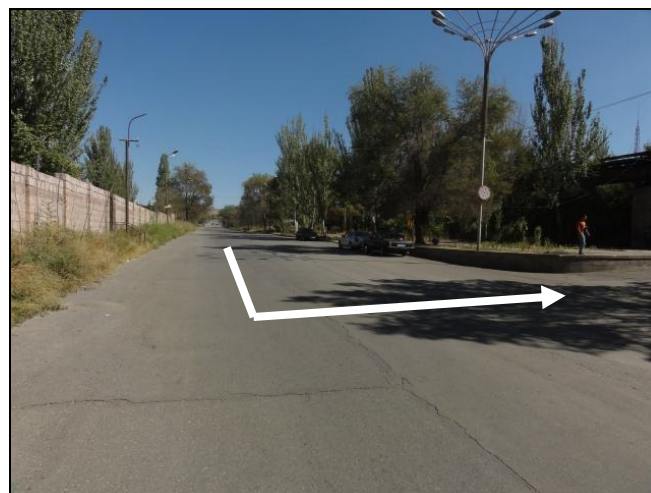
Photo 3-1: Access road to YTPC substation YTPC site
