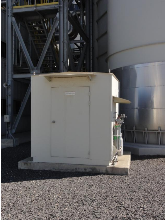
Photo 10-5: Continuous Monitoring Unit (CMS)
