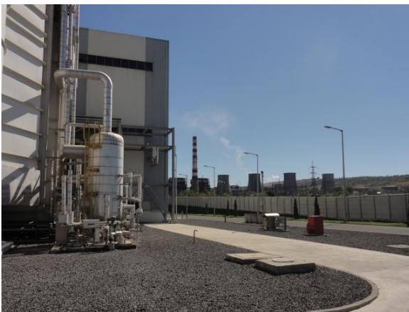
Photo 10-3: View from new to old power plant site
