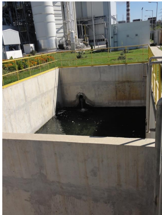
Photo 10-7: Outlet of treated process water
