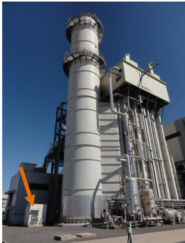
Photo 10-4: Stack with Continuous Monitoring Unit (CMS)
