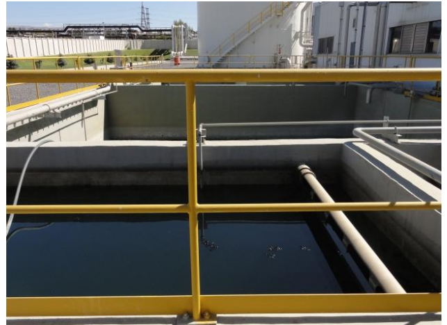
Photo 10-6: Process water treatment
