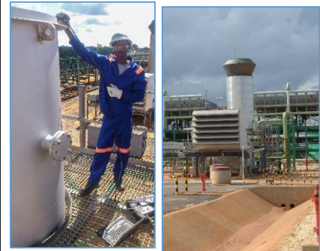
Left: Measuring emissions from the plant stacks as a basis for air pollution modelling of cumulative impacts. Right: LP Compression under construction
