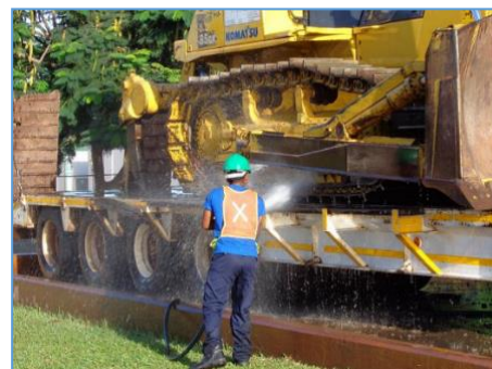
Cleaning of earth moving equipment brought into the loop line construction area for invasive plant prevention
