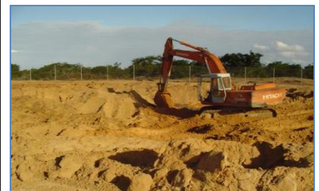
Using the mixed-bury-cover (MBC) technique to dispose of drilling waste at Inhassoro well pads
