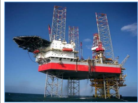
The rig on location at the Mupeji well in offshore area M-10
