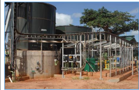
MBR (membrane bioreactor) sewage treatment plant installed at the CPF to significantly increase treatment capacity as a part of the 183 Expansion Project
