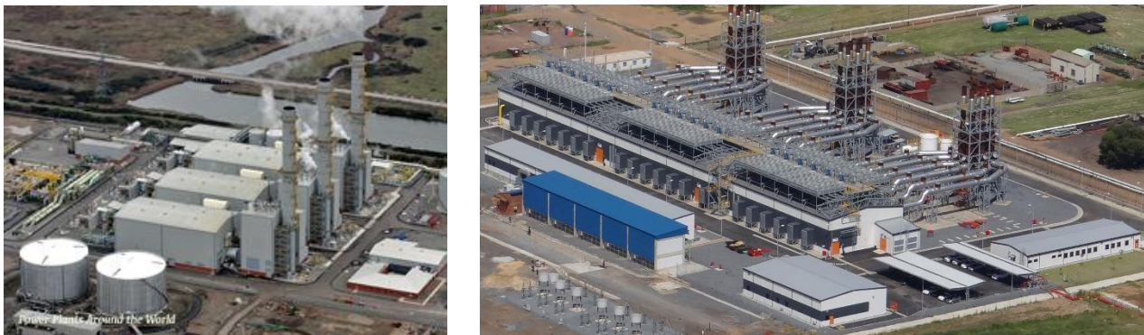
Figure 2: Examples of gas to power plant sites (source: www.industcards.com and www.wartsila.com )
