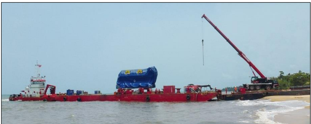
Figure 5: Example of heavy equipment being moved from the barge onto the temporary jetty using a mobile surface crane (source: Comarco)
